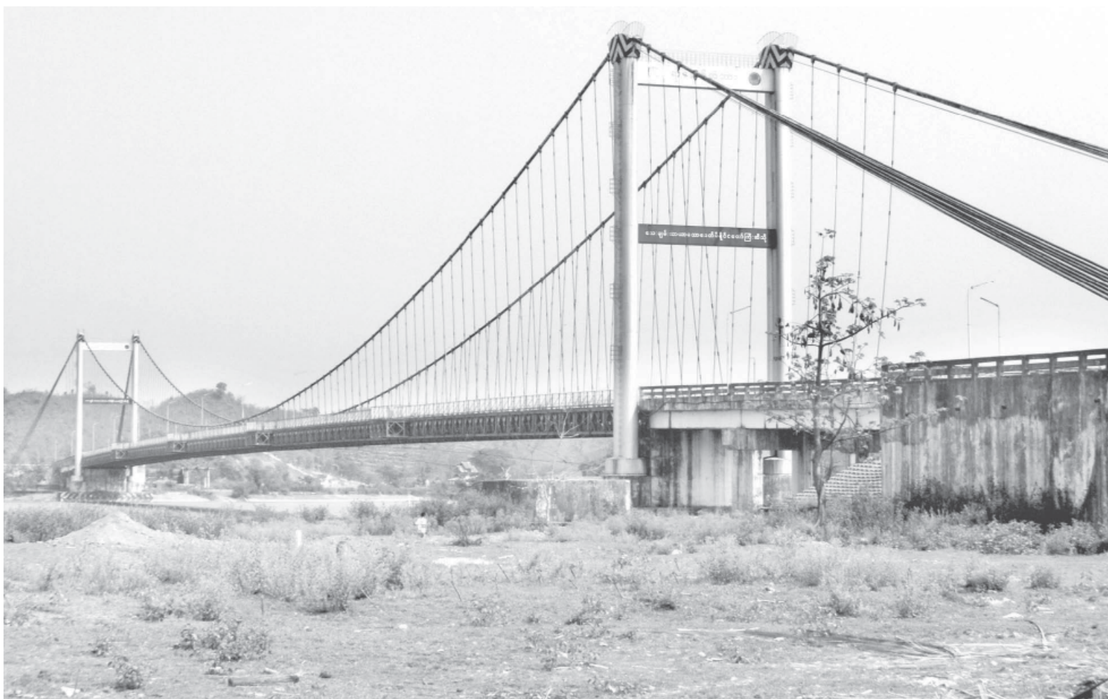
The 1300-foot-long Ya Maung Bridge on Yangon-Sittway Highway ensures smooth transport for Minbya Township.
