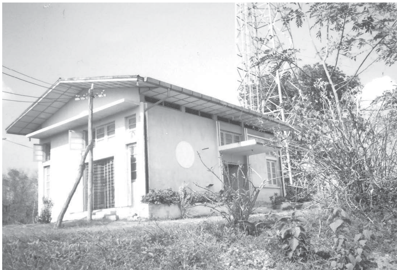
A microwave tower seen at the station of Myanma Posts and Telecommunications in Indaw Township.
