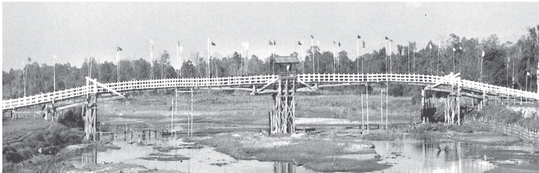
Laytan Creek Bridge linking Mahton and Mingon villages of Indaw Township.
