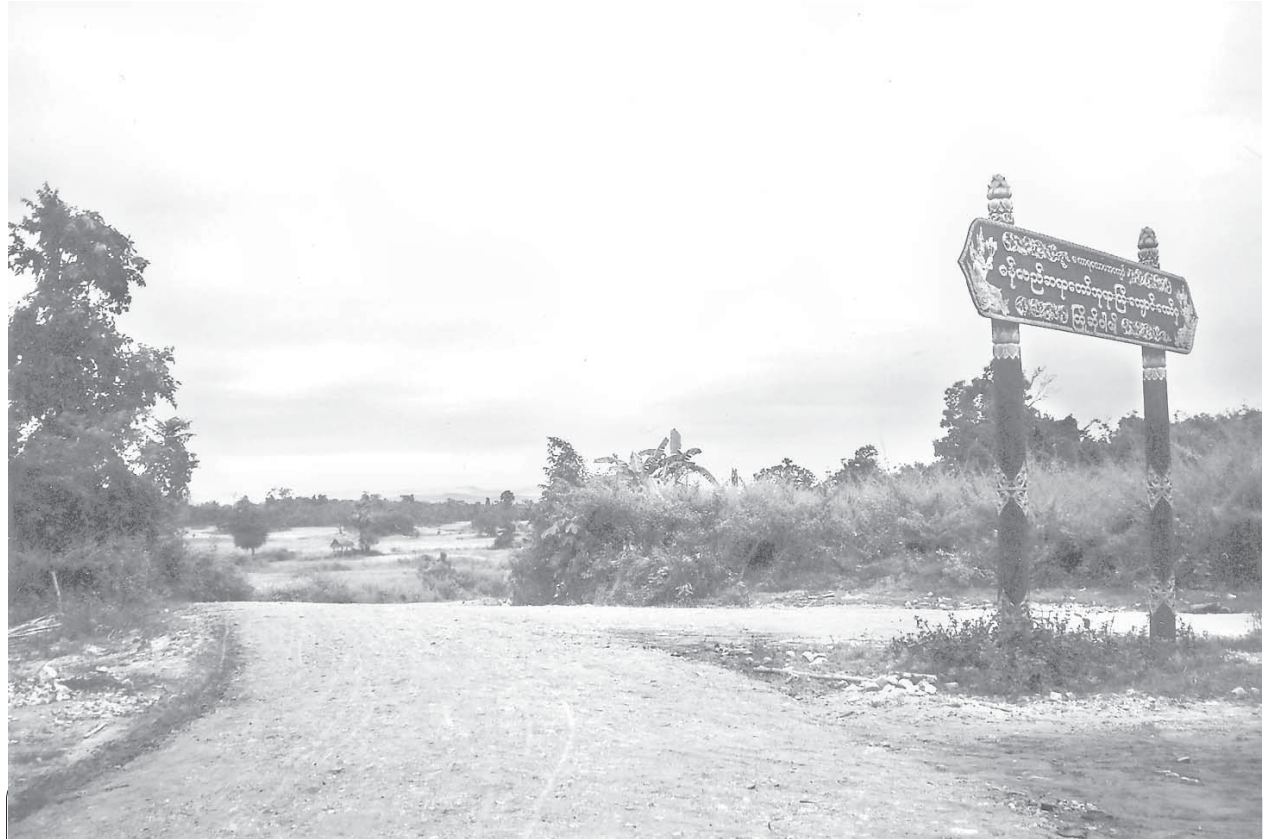
Photo shows Hseywa-Manle gravel road in Indaw Township.
