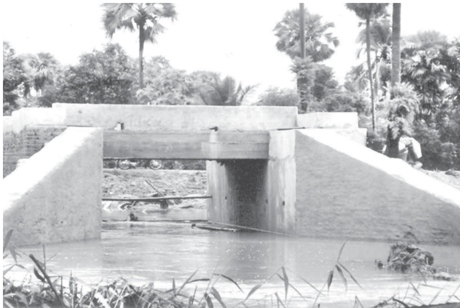
Bridge No (29) in Dawei-Thayetchaung railroad section.
