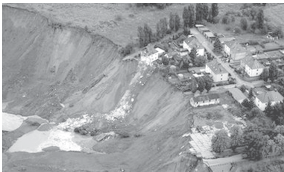
Aerial view of the area where two houses were swept away by a landslide in Nachterstedt, eastern Germany. —INTERNET
