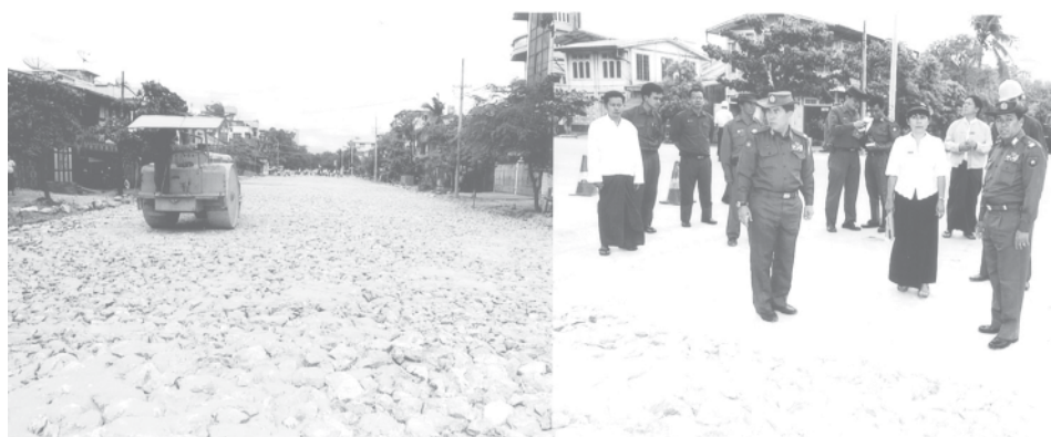
MNA Commander Maj-Gen Tin Ngwe inspects construction of road.—MNA
