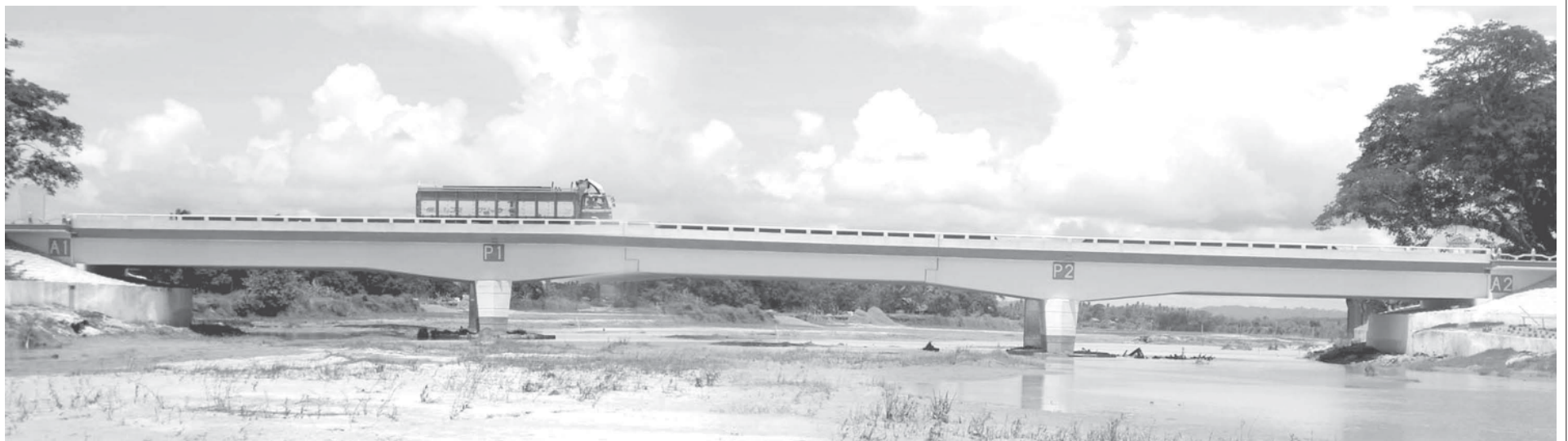
Swa Chaung Bridge spanning Swa Creek in Yedashe township.
