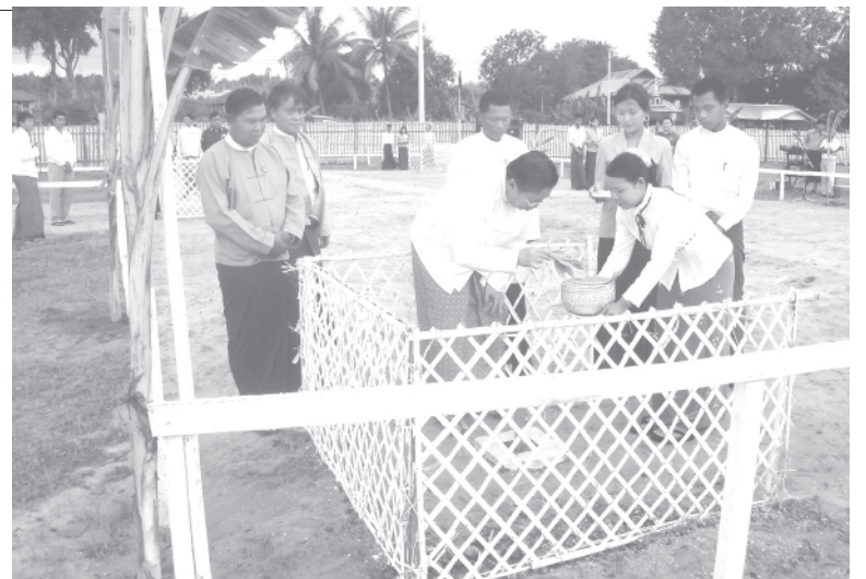
Deputy Minister Dr Paing Soe drives stake for building Myanmar Traditional Practitioners Association (Central) office. MNA
