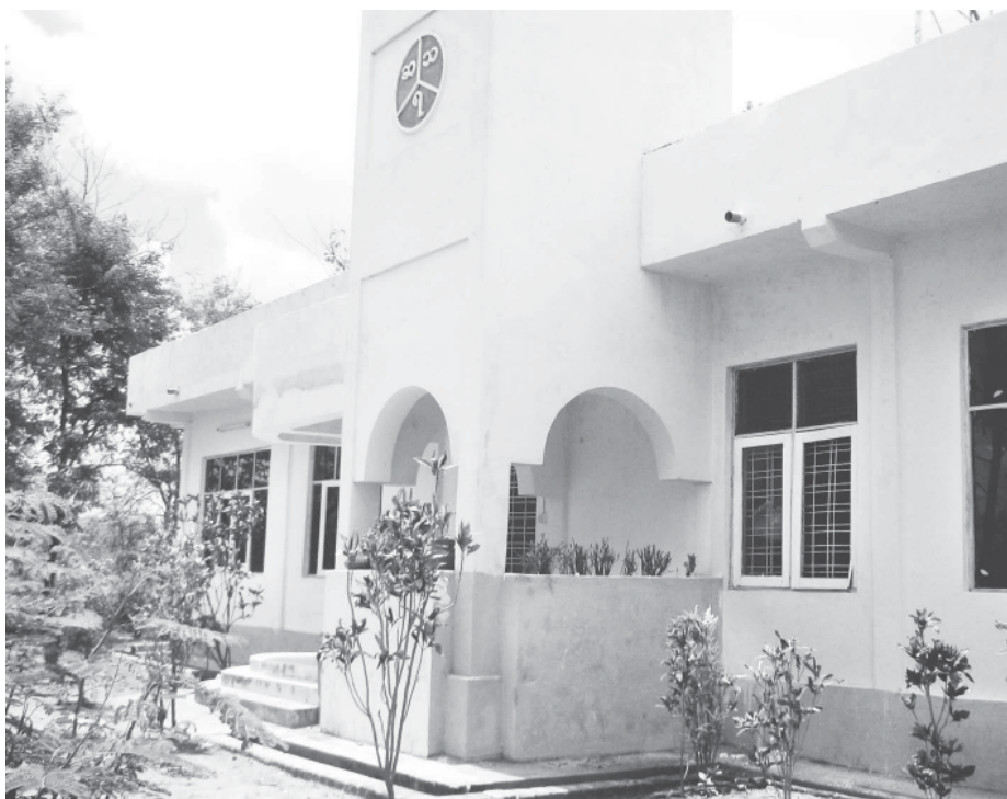
An auto-exchange built within two months in Mindon.
