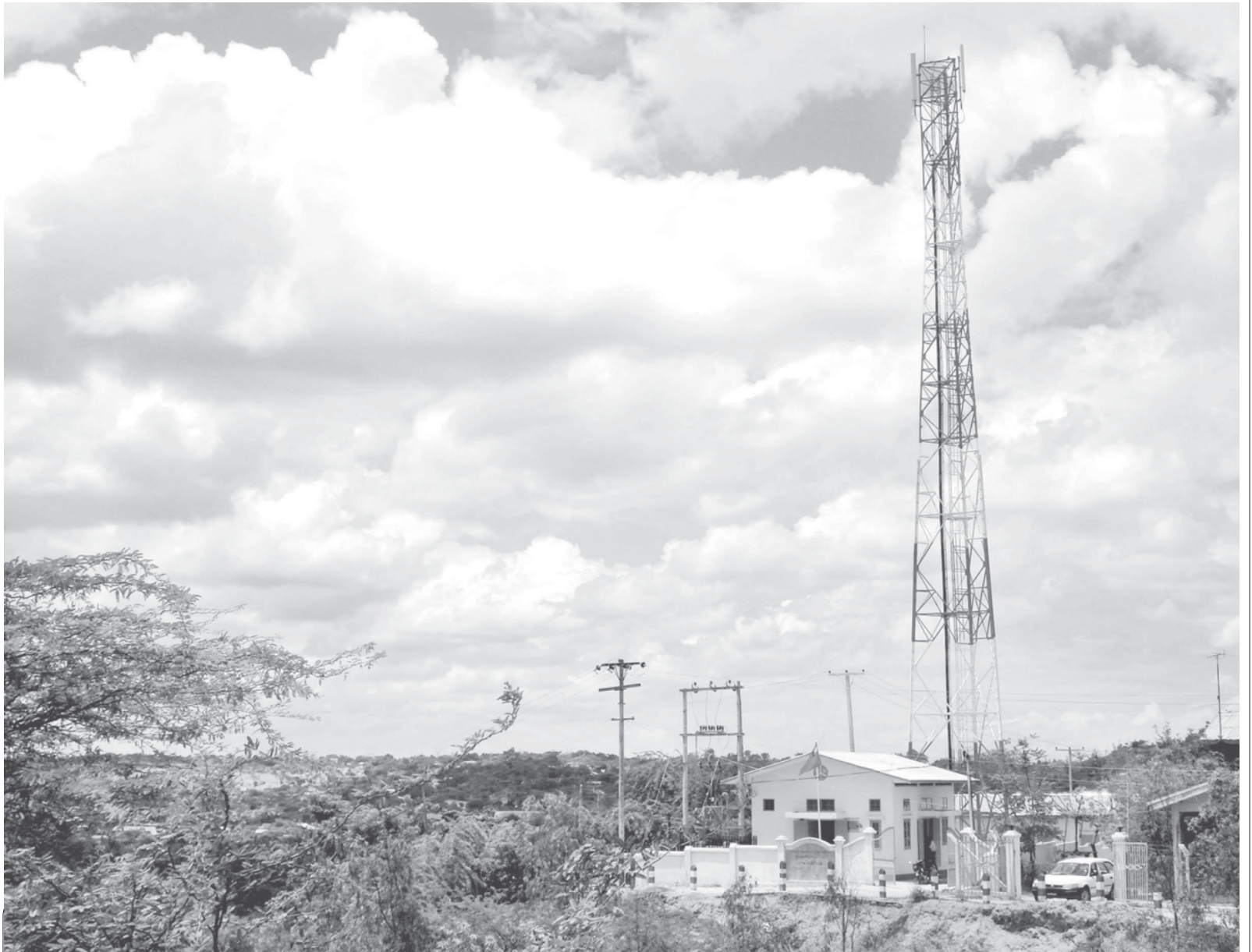
Photo shows GSM tower station in Chauk providing communication facilities to local people.
