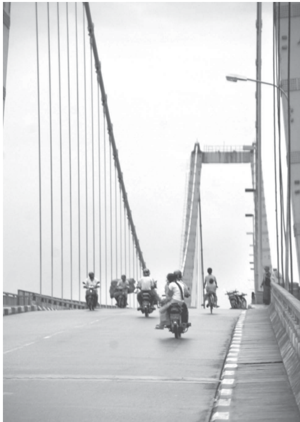
Pathein Suspension Bridge with a tarred road on it.
