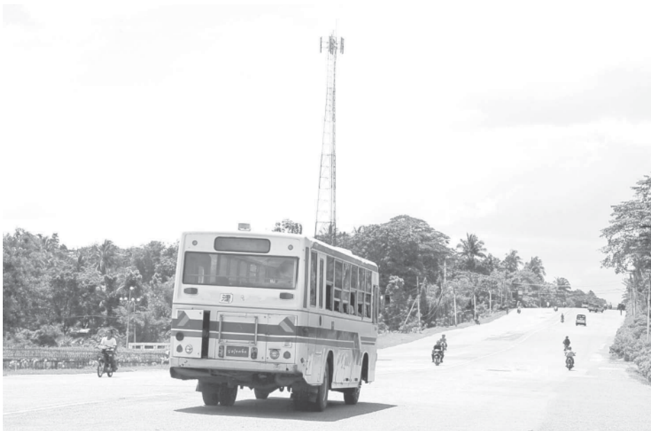
A road section (Rakhinegone) indicates significant development of Mawlamyine.
