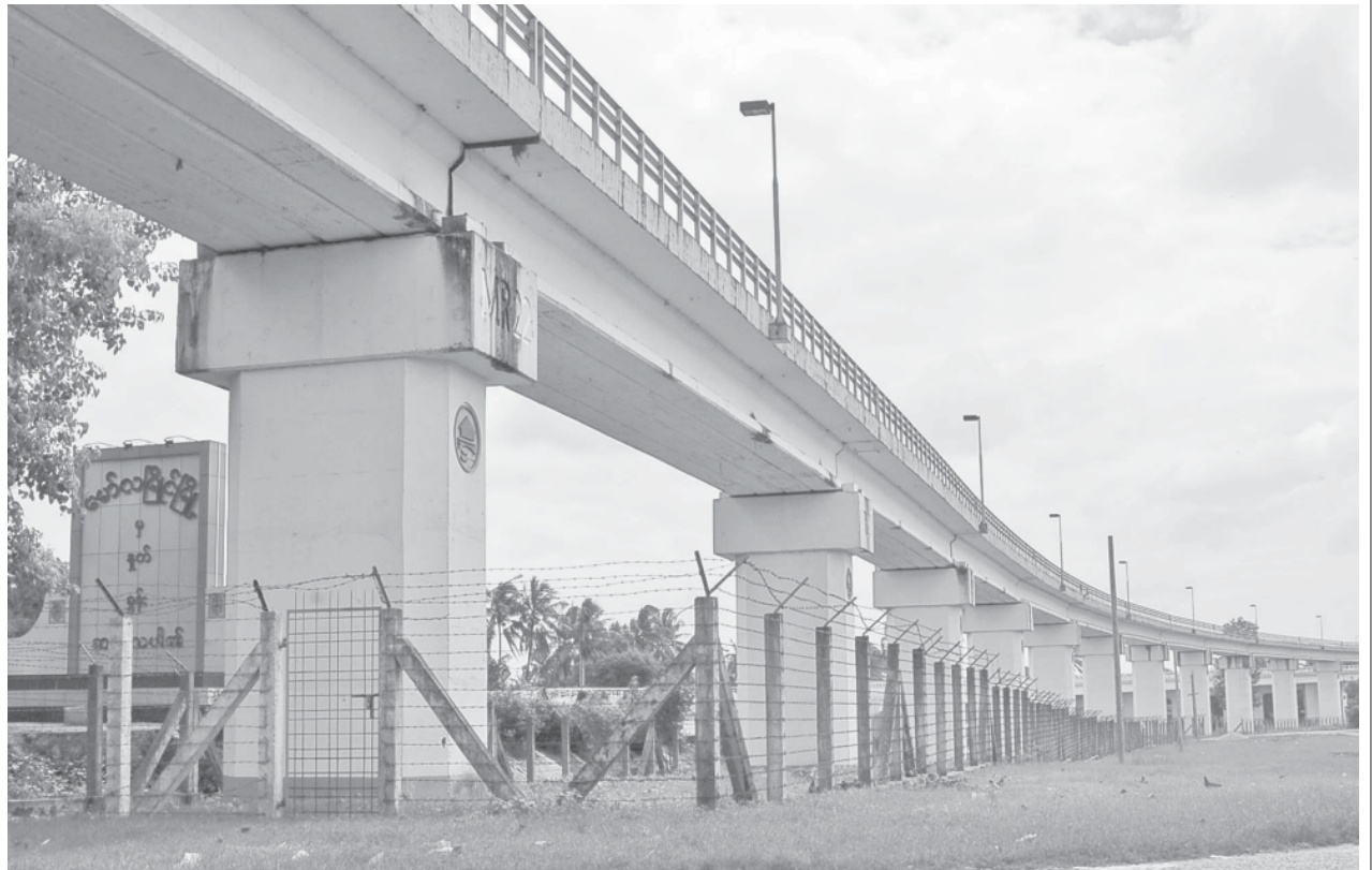
An approach road to Thanlwin Bridge (Mawlamyine).
