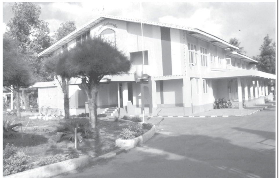
Photo shows two-storey Kandaw Mingala Hall in Meiktila.
