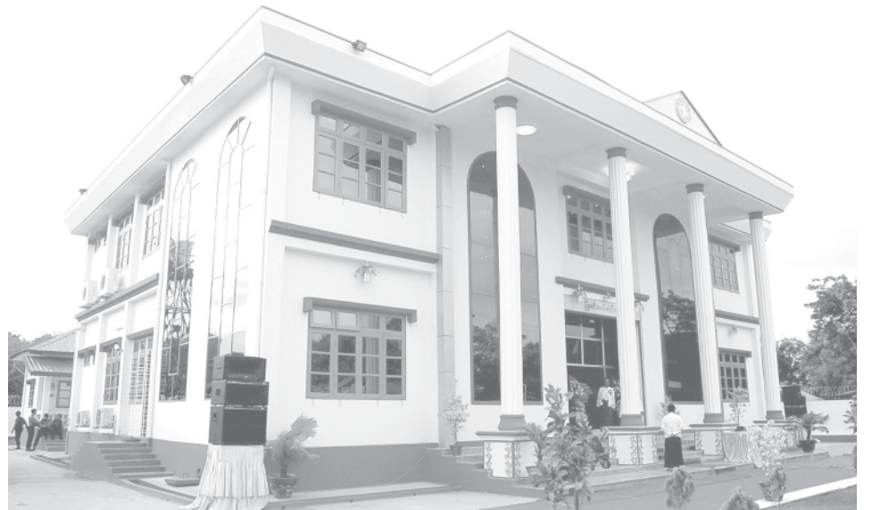
Photo shows new building of Myawady Bank Ltd (Pyawbwe).
