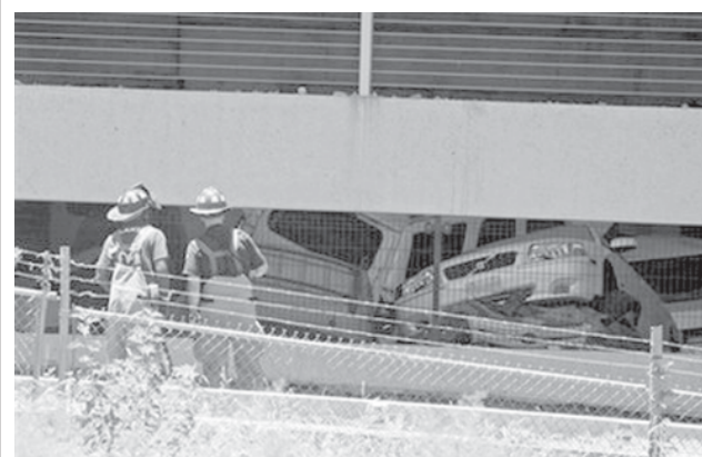
Firefighters look at damaged vehicles in a collapsed garage in Atlanta, on 29 June, 2009. Part of a six-floor parking deck at a building near downtown Atlanta collapsed crushing dozens of cars, but there were no immediate reports of injuries.—INTERNET
