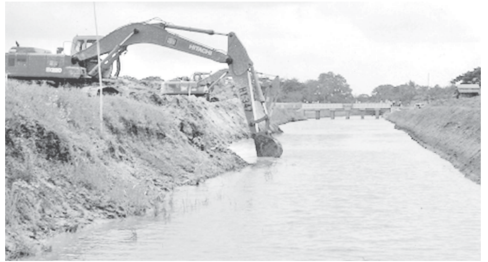
An excavator at work at Thakala-Kayan section.
