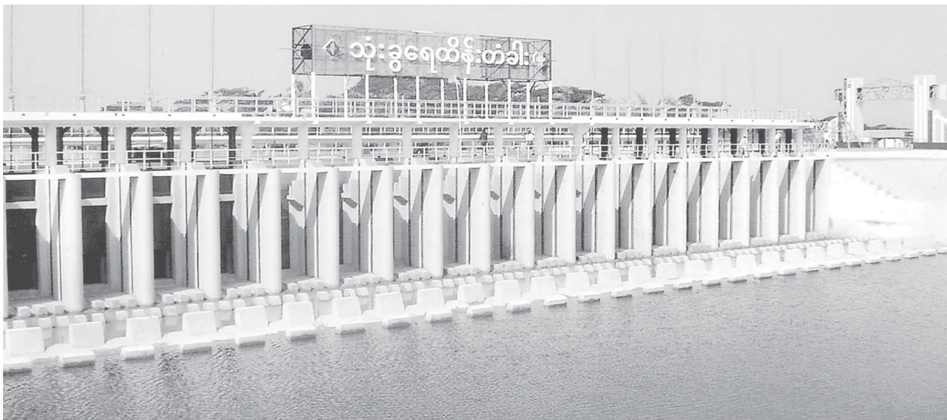
Thongwa Sluice Gate designed to contribute towards Project for Greening 30-mile Radius of Yangon.
