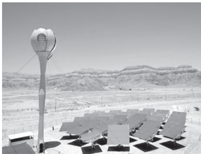
Photo taken on 24 June, 2009 shows the solar receiver of the world's first hybrid solar thermal power station at Kibbutz Samar in southern Israel. XINHUA
