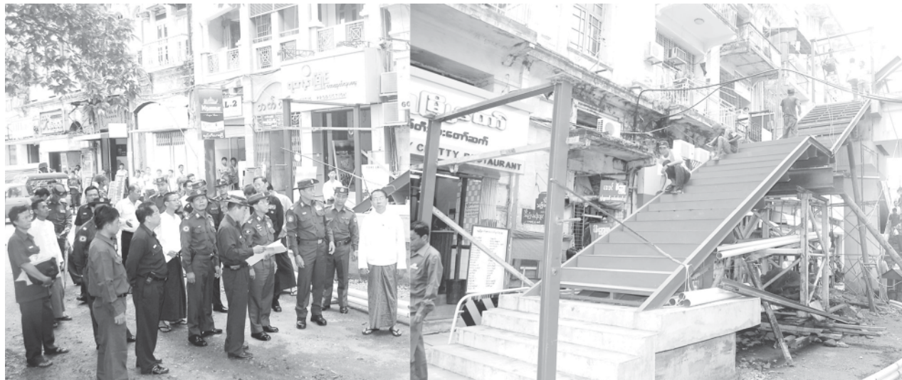
Lt-Gen Myint Swe of Ministry of Defence looks into maintenance of Tawwin overpass in Kyauktada Township.—MNA
