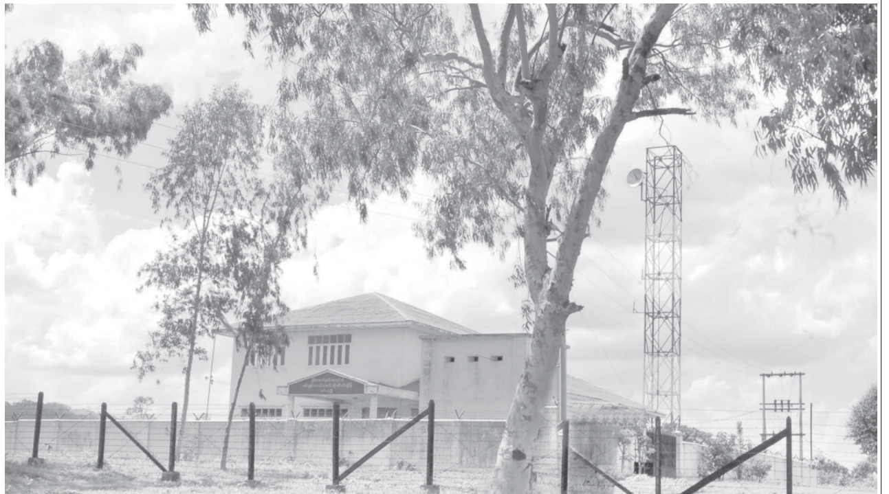
Digital auto exchange of the Myanmar Posts and Telecommunications in Loilem Township.
