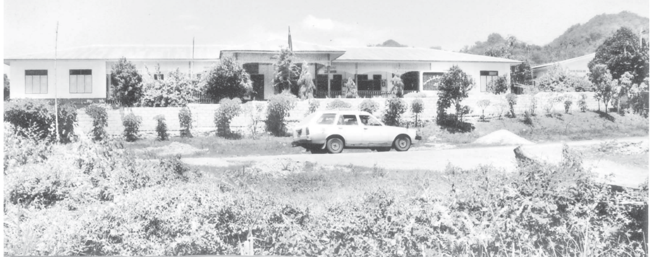
The 16-bed station hospital in Sanlaung Village, Hsenwi Township.
