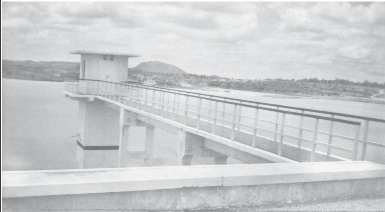
Water control tower seen at Gwegyo Dam.
