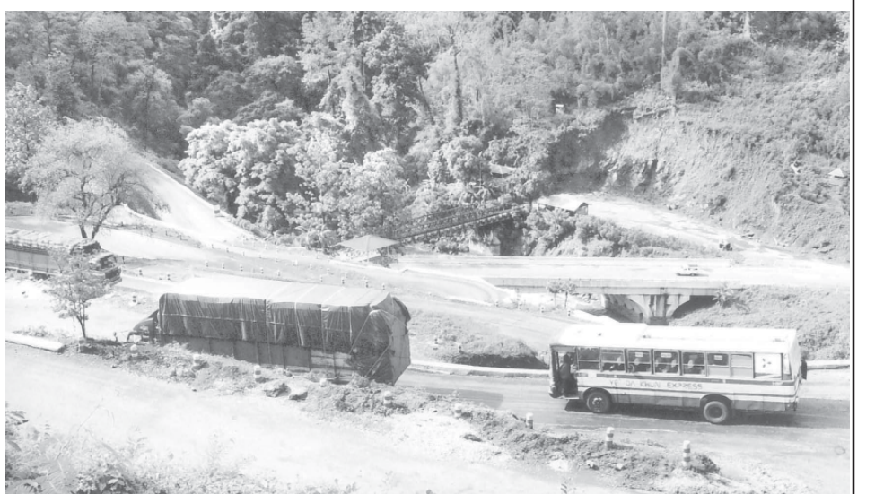
The motor road zig-zags near Goktwin Bridge in Nawngkhio Township.
