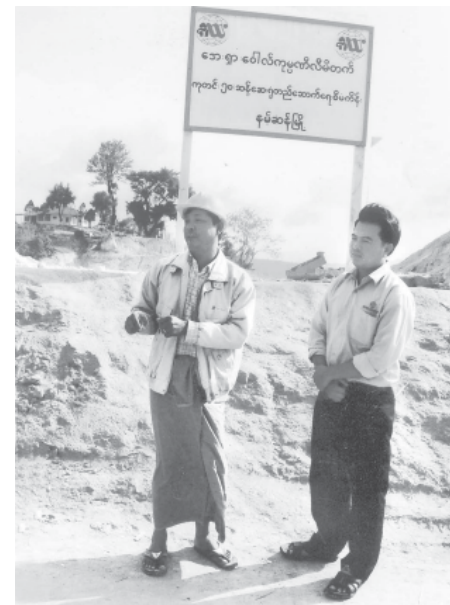
Completion of the whole project by October 2009 is on target. (U San Maung (left), in-charge of Namsang People's Hospital (50-bed) Project construction site.
