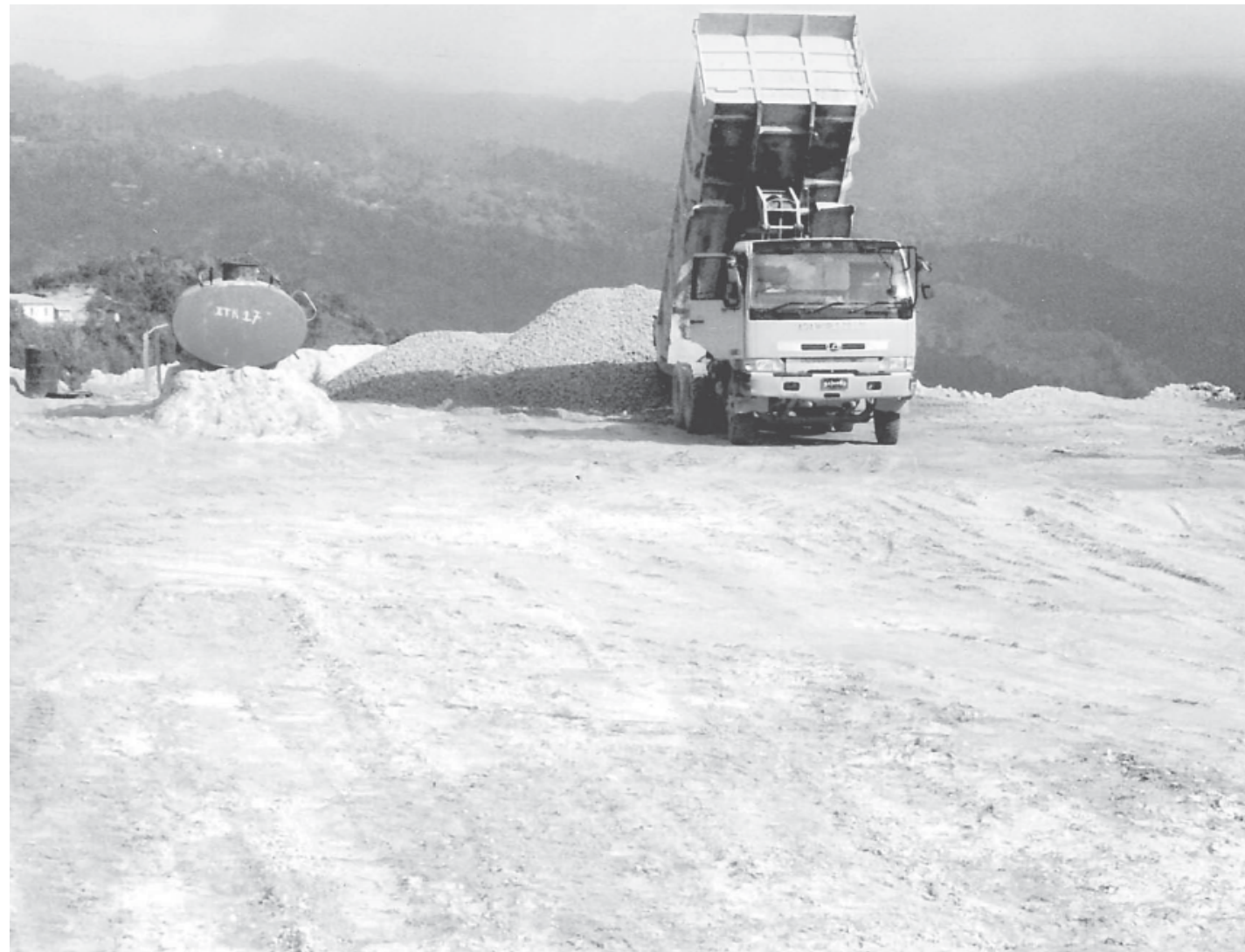
A tipper lorry carrying out groundwork at work site.
