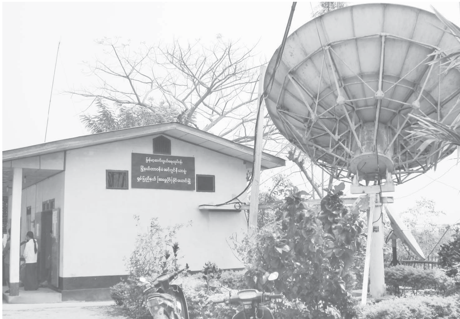
Office of the township engineer-in-charge and satellite station seen in Mongyawng.
