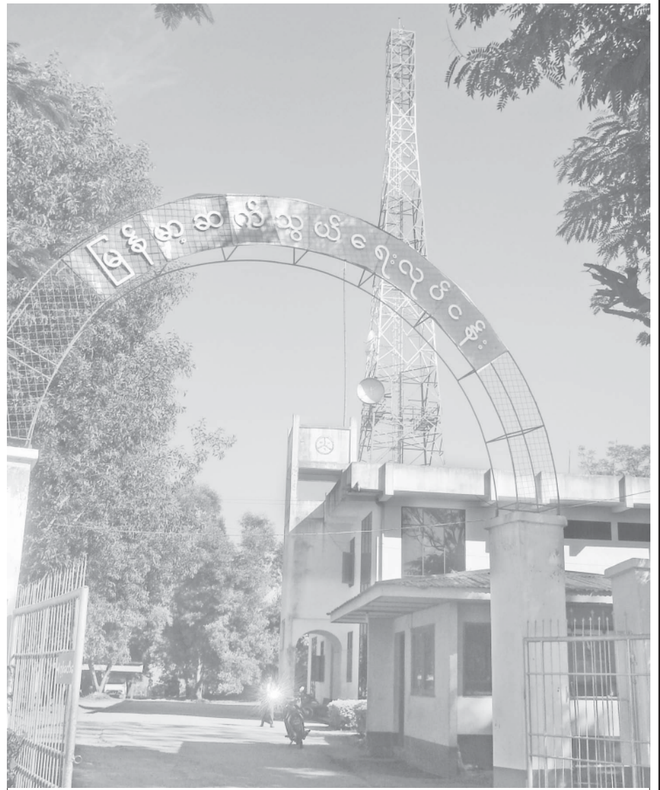
Myanma Posts and Telecommunications Office and a microwave tower seen in Kengtung of Shan State (East).
