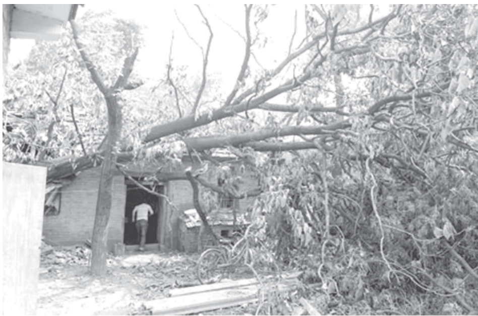
The house of Zhang Xiulin, a farmer of Shilipu village, is destroyed by a big fallen tree after the strong storm and rain swept Shangqiu, east China’s Henan Province, 5 June, 2009. Strong storm, gales, hailstones and heavy rain whipped Shangqiu on Wednesday, leaving at least 20 people dead and 79 injured.—XINHUA
