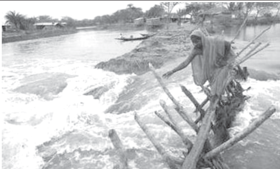
A woman crosses a bamboo made bridge over a breached dam caused by cyclone Aila in Shatkhira on 4 June, 2009. Thousands of people have been displaced by a huge tidal wave caused by cyclone Aila on May 25. Survivors are suffering due to scarcity of food and drinking water.—INTERNET
