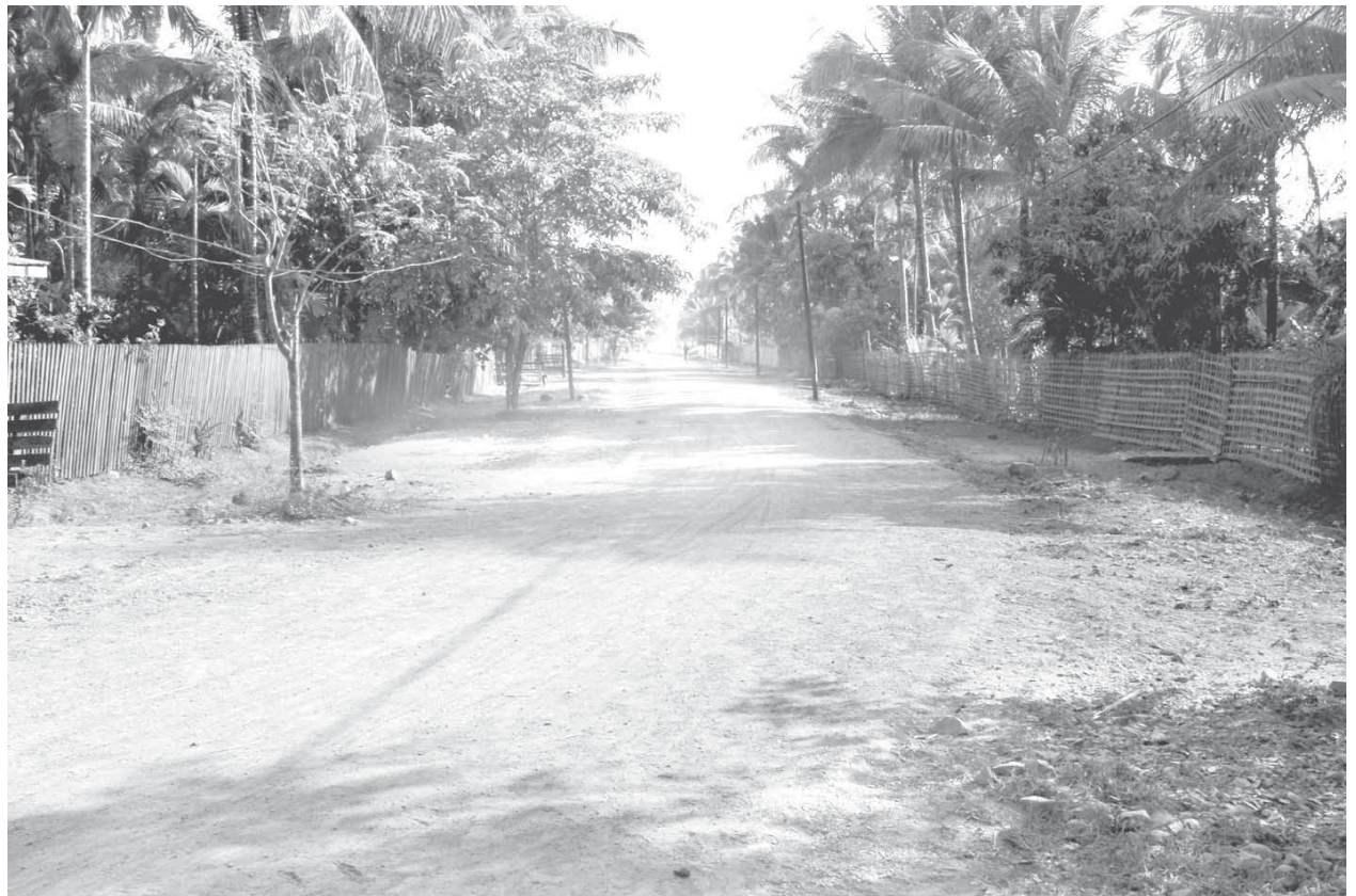
U Uttama Road seen after being renovated.
