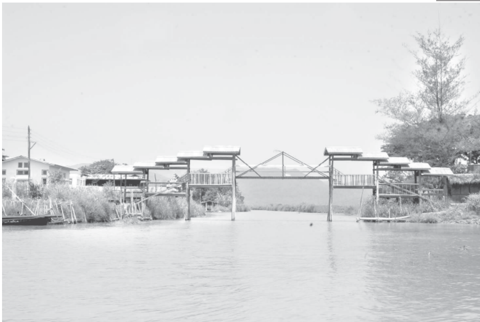
A bridge linking villages seen in Inlay Lake.
