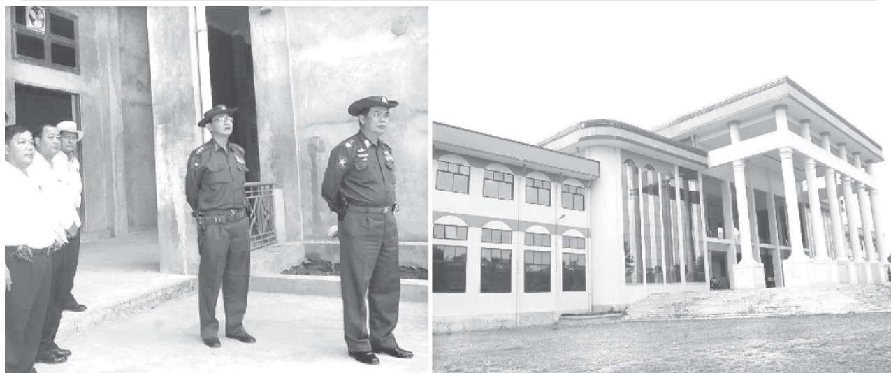
Lt-Gen Tha Aye views construction of main building at Magway University.
