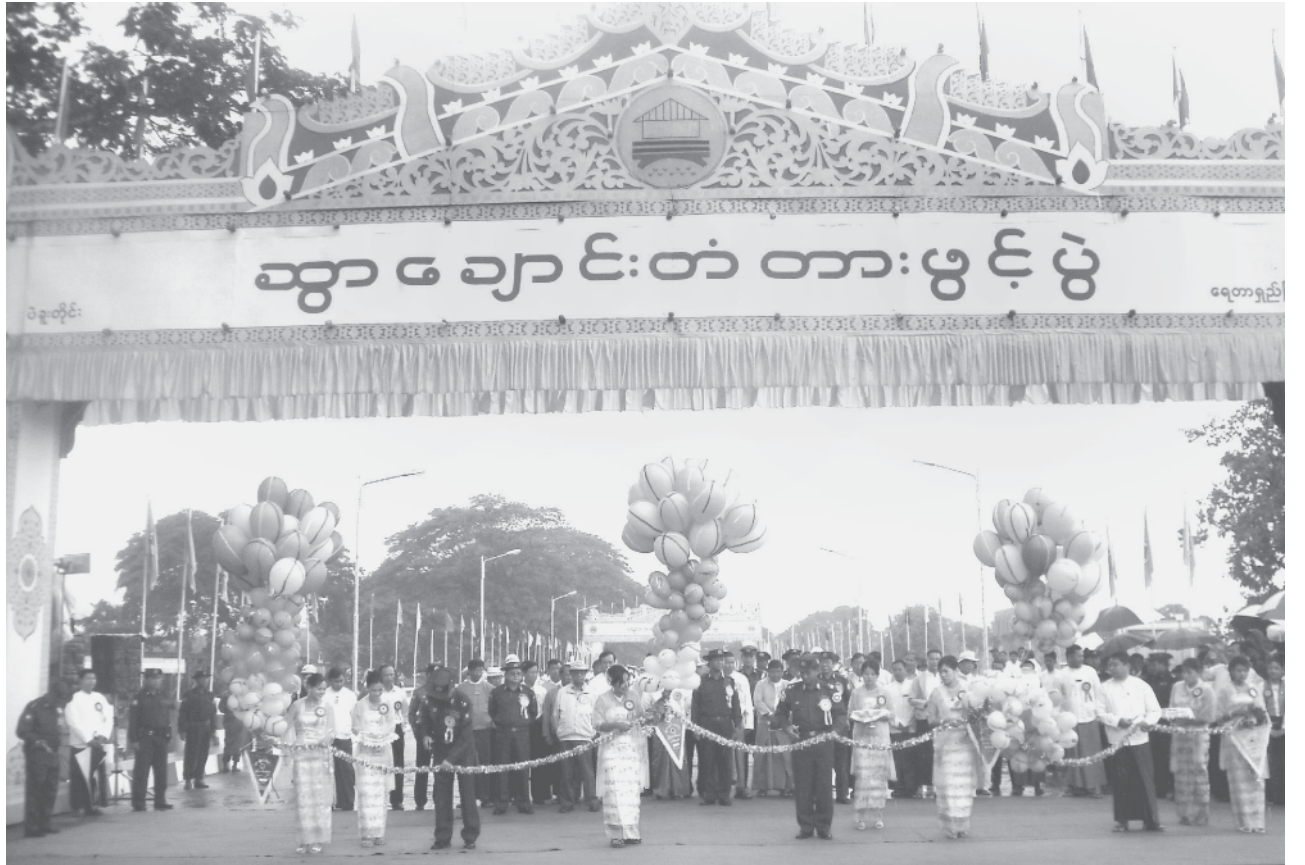
Ministers Maj-Gen Khin Maung Myint and Maj-Gen Aung Min cut the ribbon to open Swa Creek Bridge.—MNA
