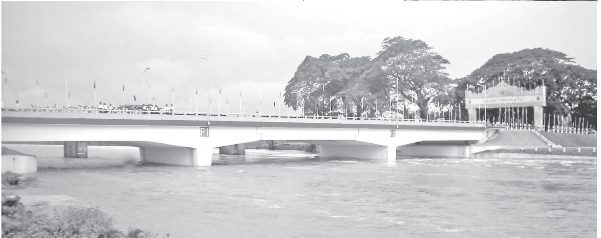
Newly-opened Swa Creek Bridge in Yedashe Township.—MNA
