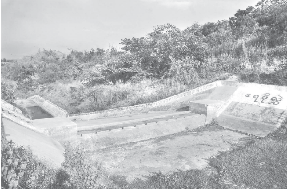
The spillway of Thebyu Dam.
