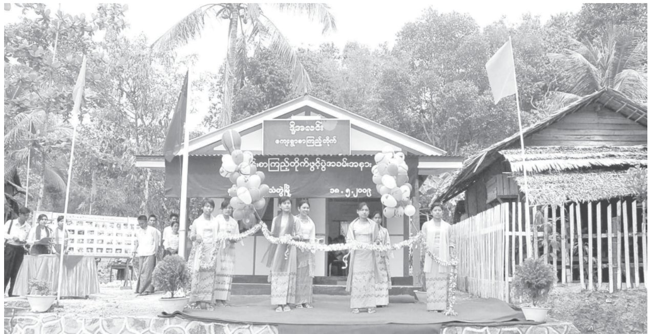
Opening of Doh Alin Library in Nanchaung Village, Thandwe, Rakhine State, in progress on 18-5-2009.
