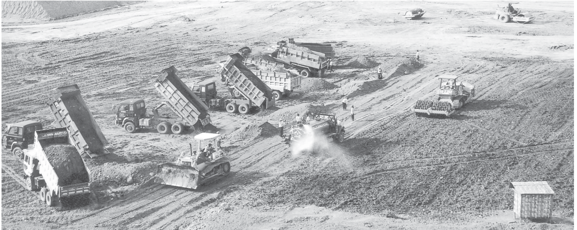
Tipper lorries, bulldozers and compactors operating for groundwork.
