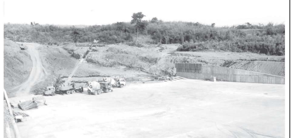
On completion, the spillway will be 991 feet long and 250 feet wide.
