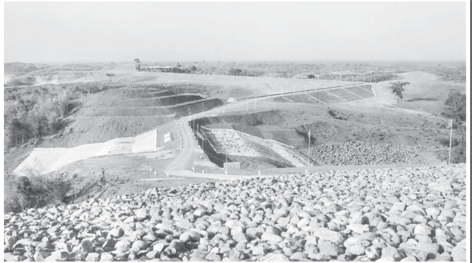
Dykes 2, 3 and 4 of Kanyin Dam Project in Ingapu Township, Ayeyawady Division.
