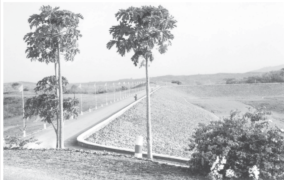
The main dam of Kanyin Dam in Ingapu Township, Ayeyawady Division.
