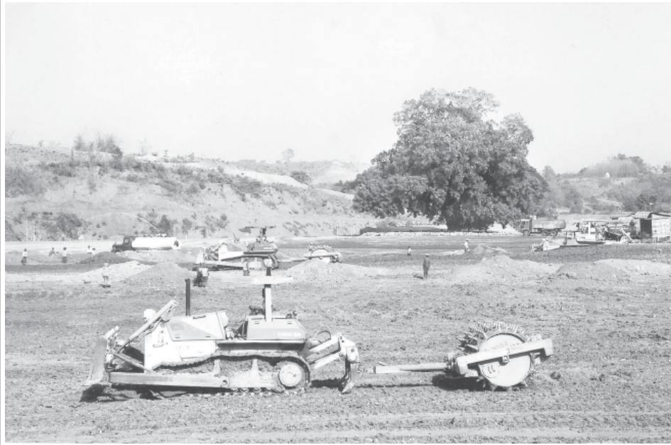
Groundwork is done with heavy machinery.
