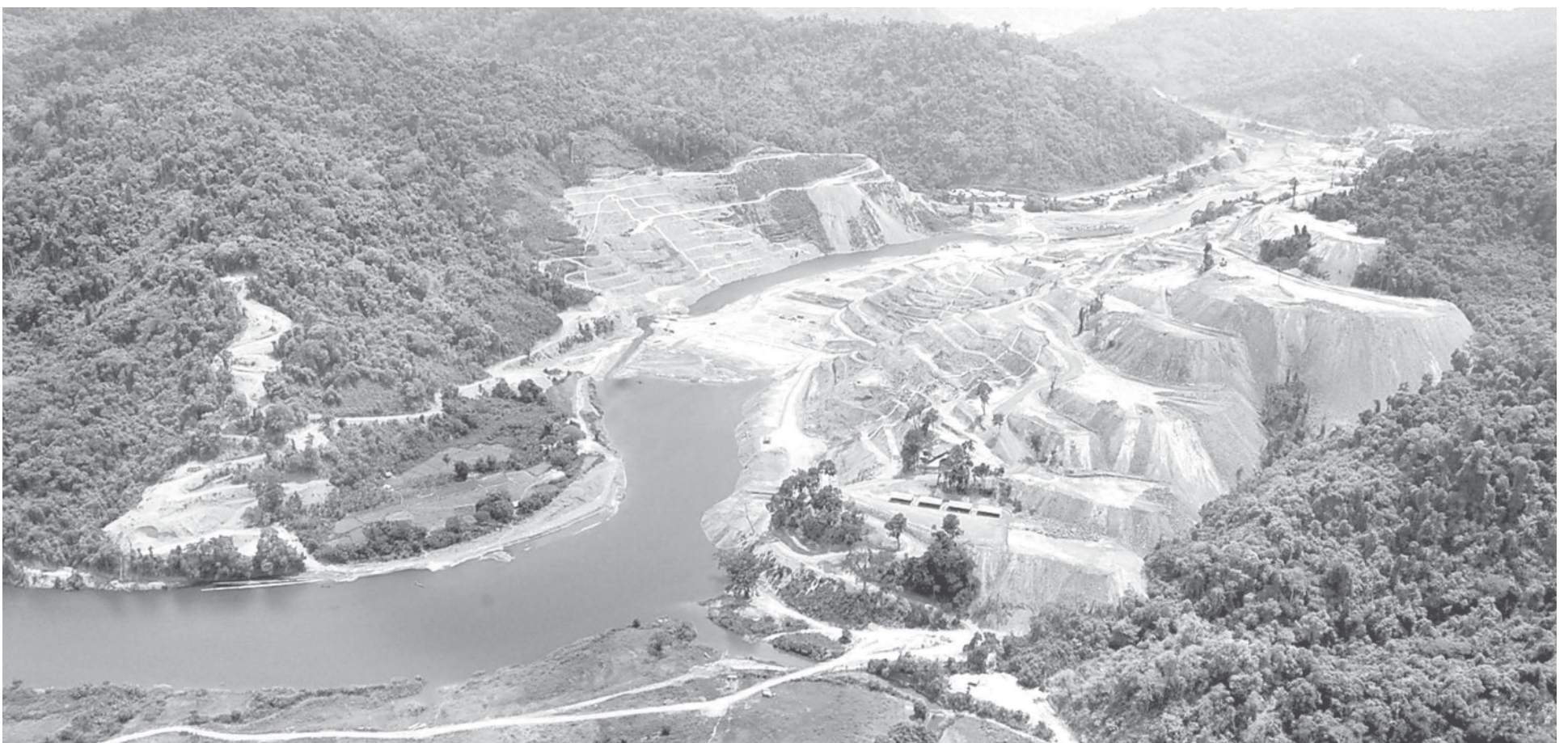
Thahtay Hydro Power Project Site.—MNA
