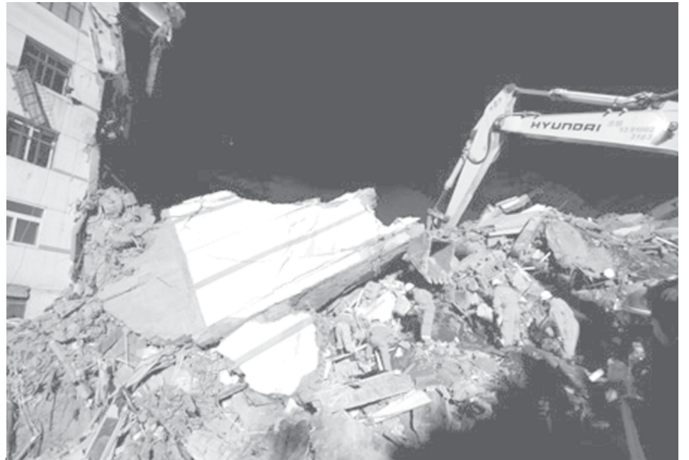
Rescuers search for survivors on the spot of a collapsed building at the Jiuzhou Economic Development Zone in Lanzhou, capital of northwest China's Gansu Province, on 17 May, 2009. Part of the residence building collapsed due to a landslide on late Saturday in Lanzhou. The bodies of two victims have been found in the scene and one injured was rescued.—INTERNET
