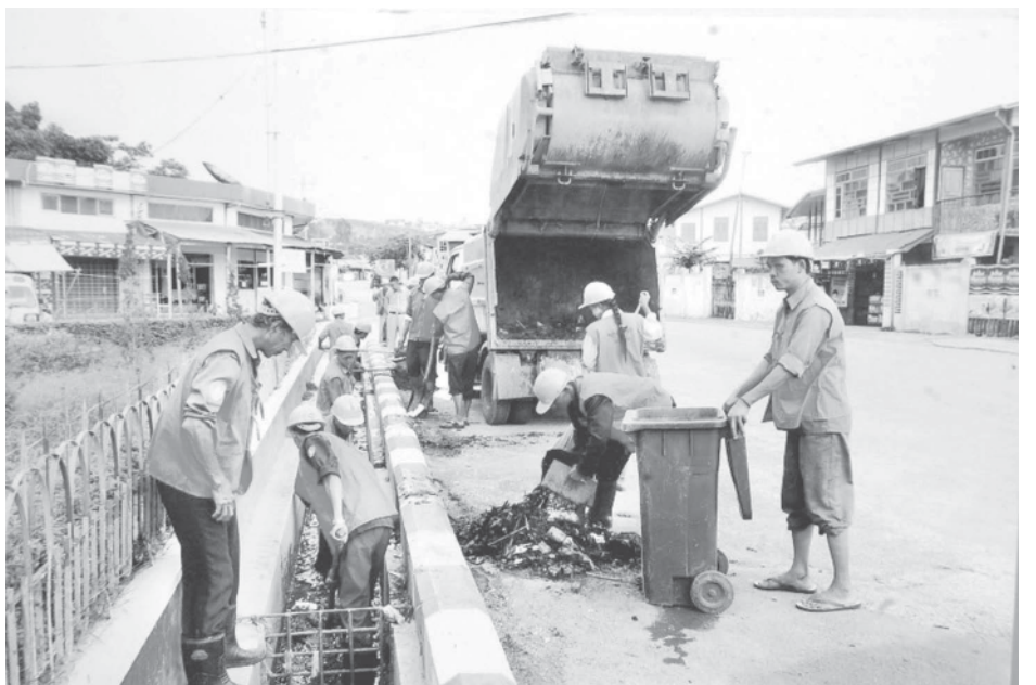
Workers dredging a drain in downtown Taunggyi.
