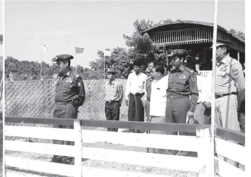
Lt-Gen Tha Aye of the Ministry of Defence inspects construction of Mya Sanda bridge and retaining wall in Homalin.—MNA
