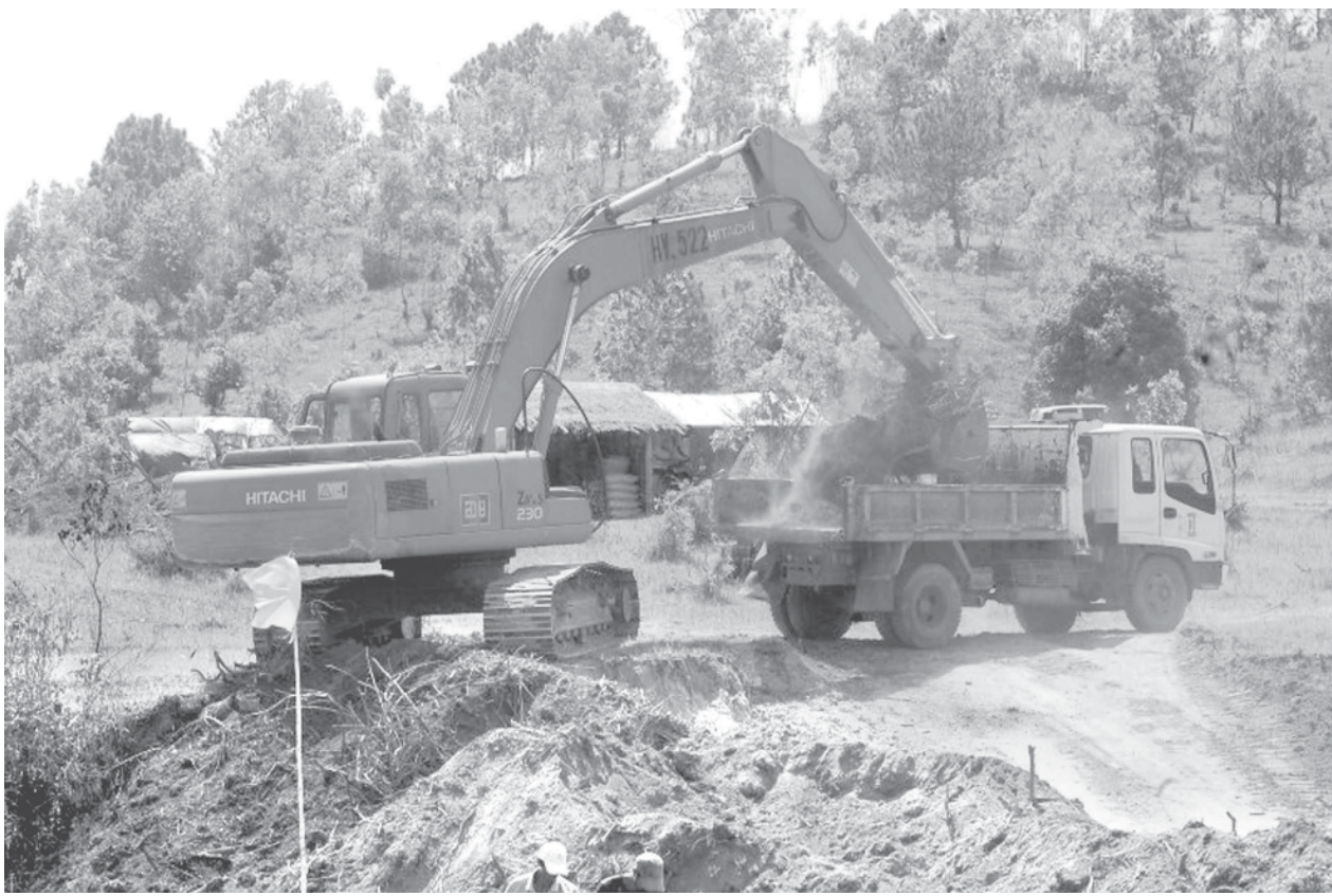
Heavy machinery being used at construction of Htithein Water Supporting Dam.
