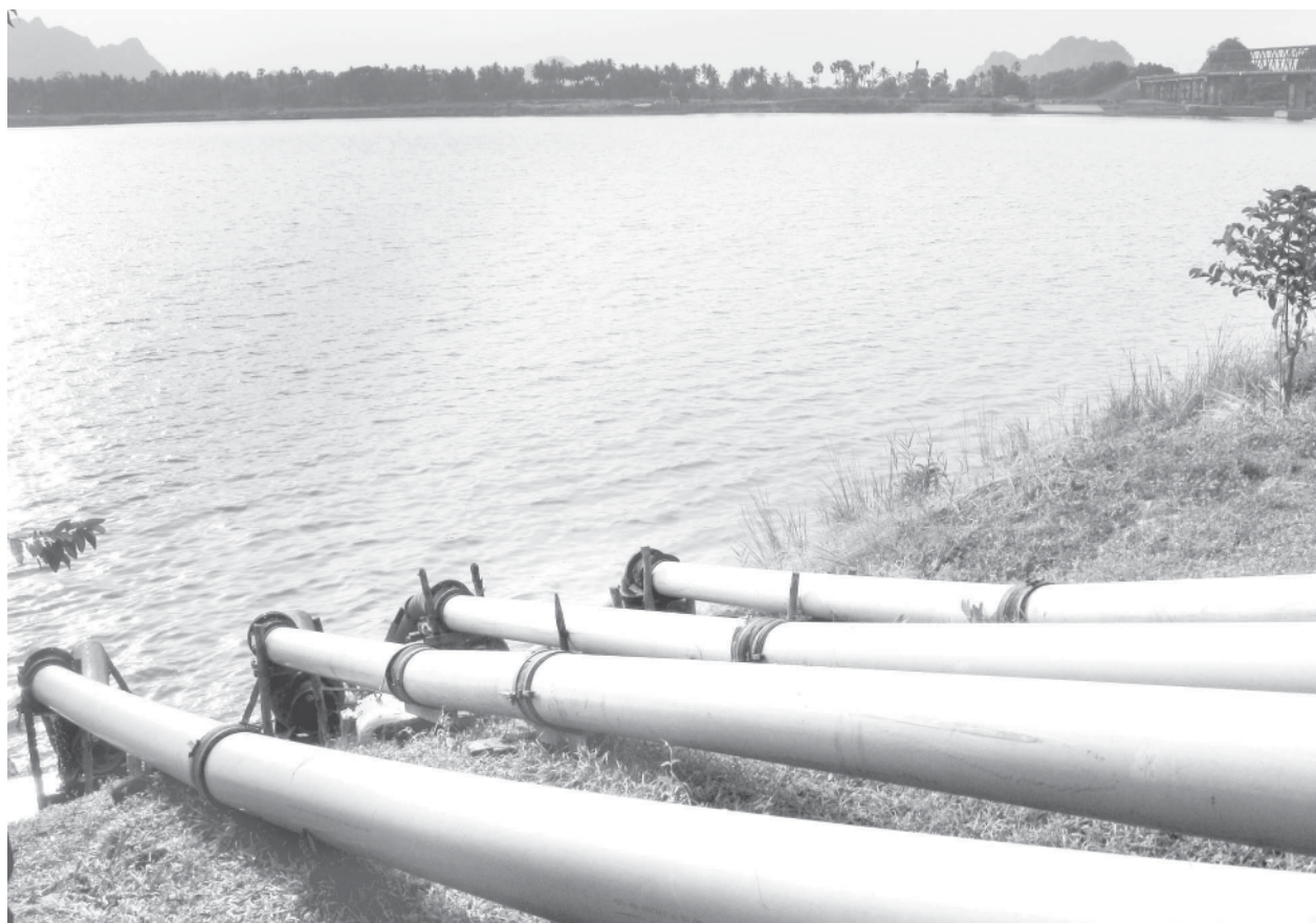
Water being pumped from Thanlwin River through four large pipes.
