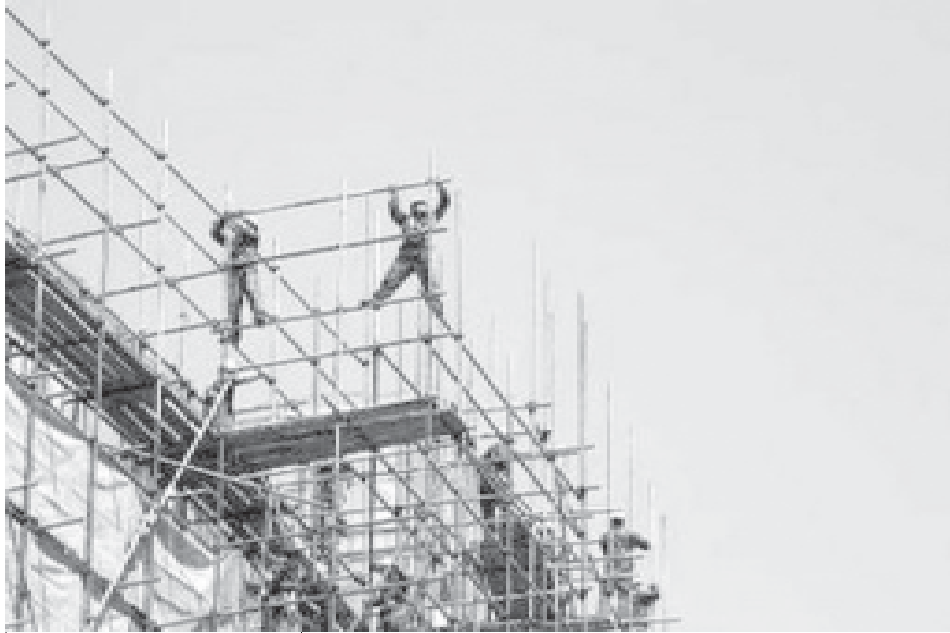
Workers install a scaffolding outside a building for a renovation in Beijing, on 13 May, 2009. Chinese real estate investment rose 4.9 percent in the first four months of 2009 from the same period a year earlier, the National Bureau of Statistics said on Tuesday, the latest sign of a gradual recovery in the sector.
