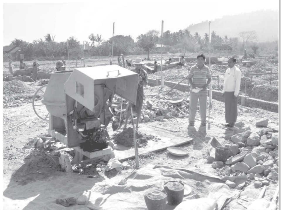
Hsarchet Station Hospital Project site in Manaung Township.
