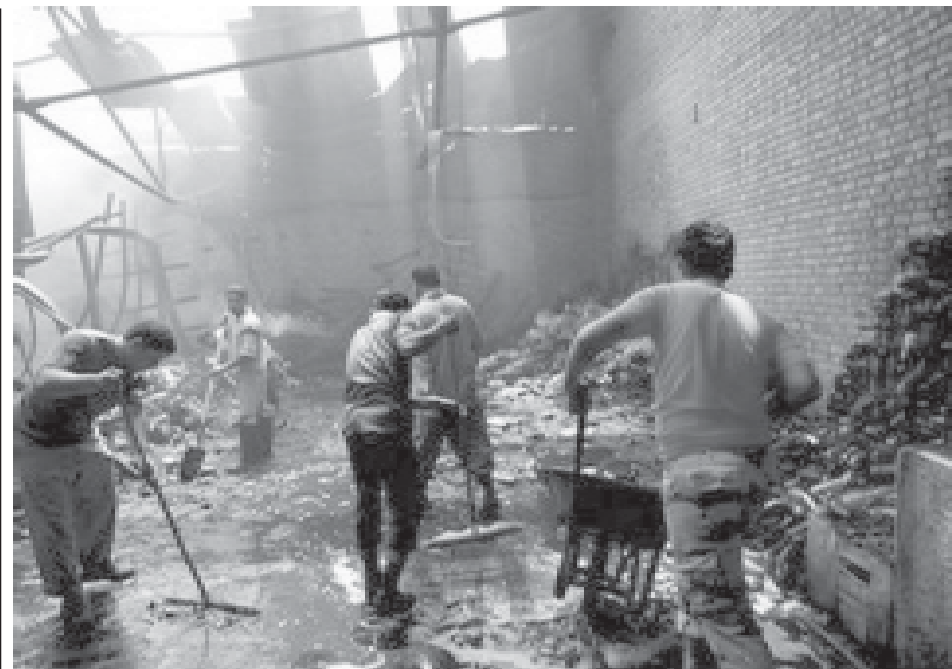
Men clean up at a warehouse heavily damaged in a fire in Basra, Iraq, on 11 May, 2009. A huge fire erupted at a wholesale market in central Basra Sunday night, damaging as many as twenty different warehouses.—INTERNET
