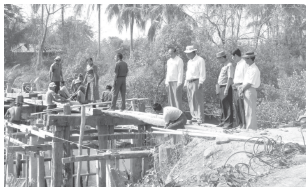
Those responsible supervise construction of 130 feet long Panchaung Bridge.
