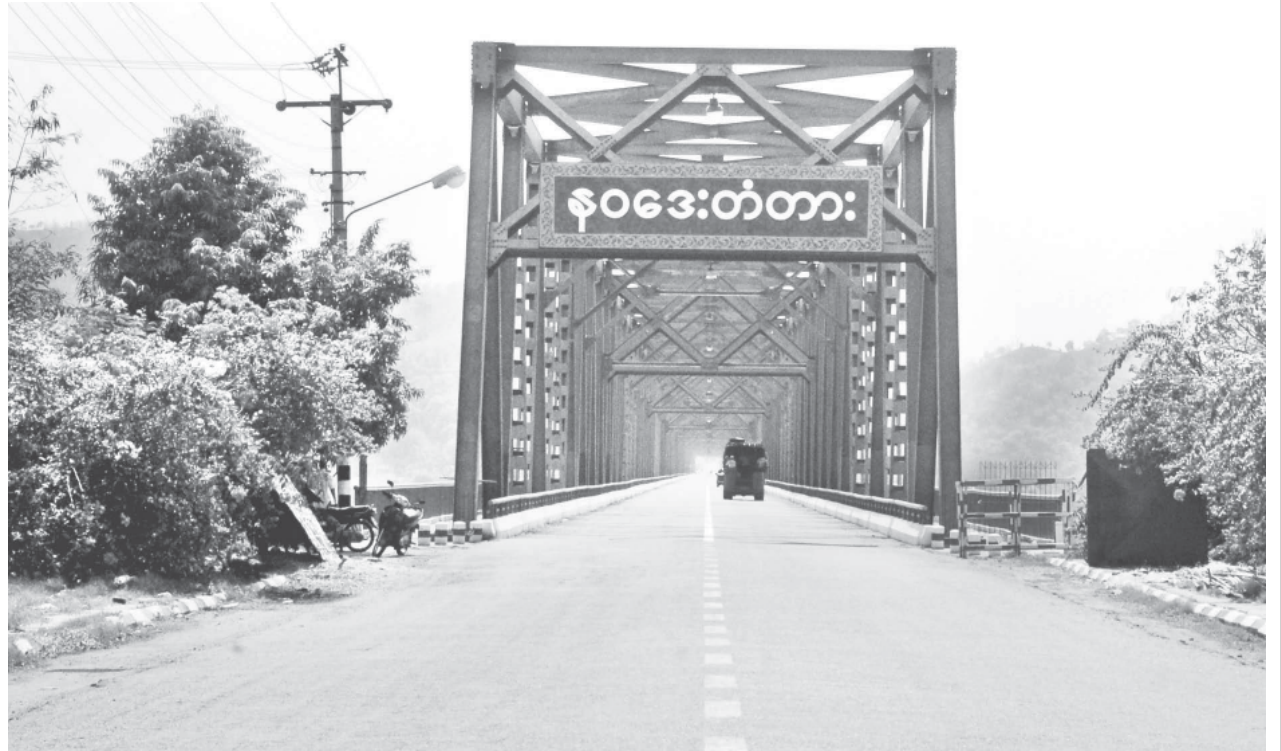
The approach road to Nawaday Bridge on Pyay side.
