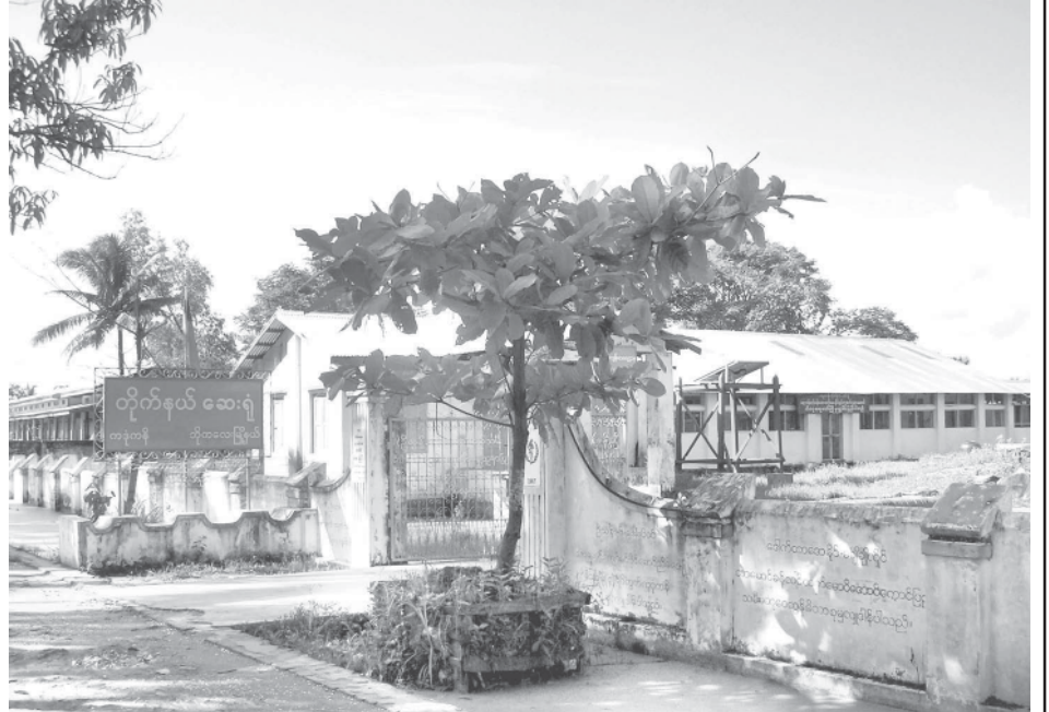
Photo shows newly renovated Kadonkani Station Hospital in Pyapon District.
