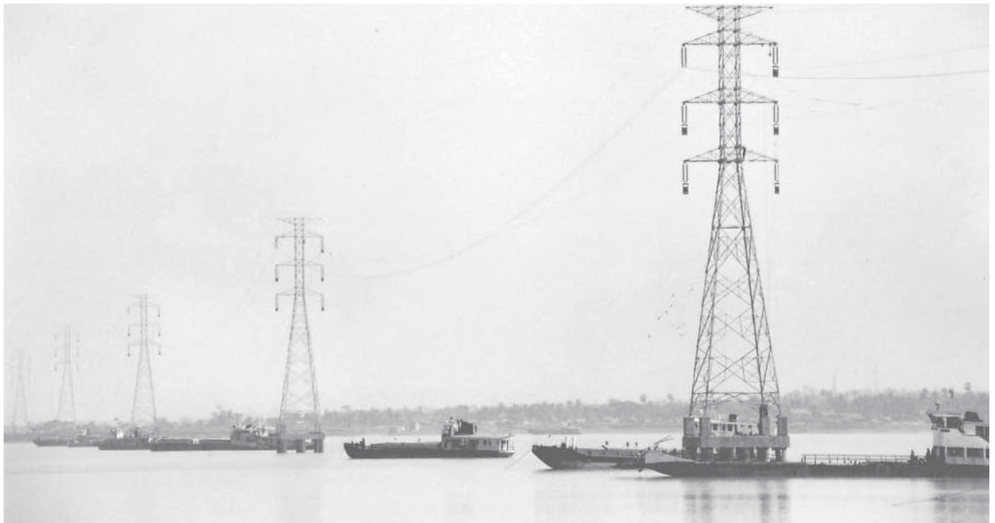
Pylons are being set up across the Bago River on 19 February 2009.—MNA
