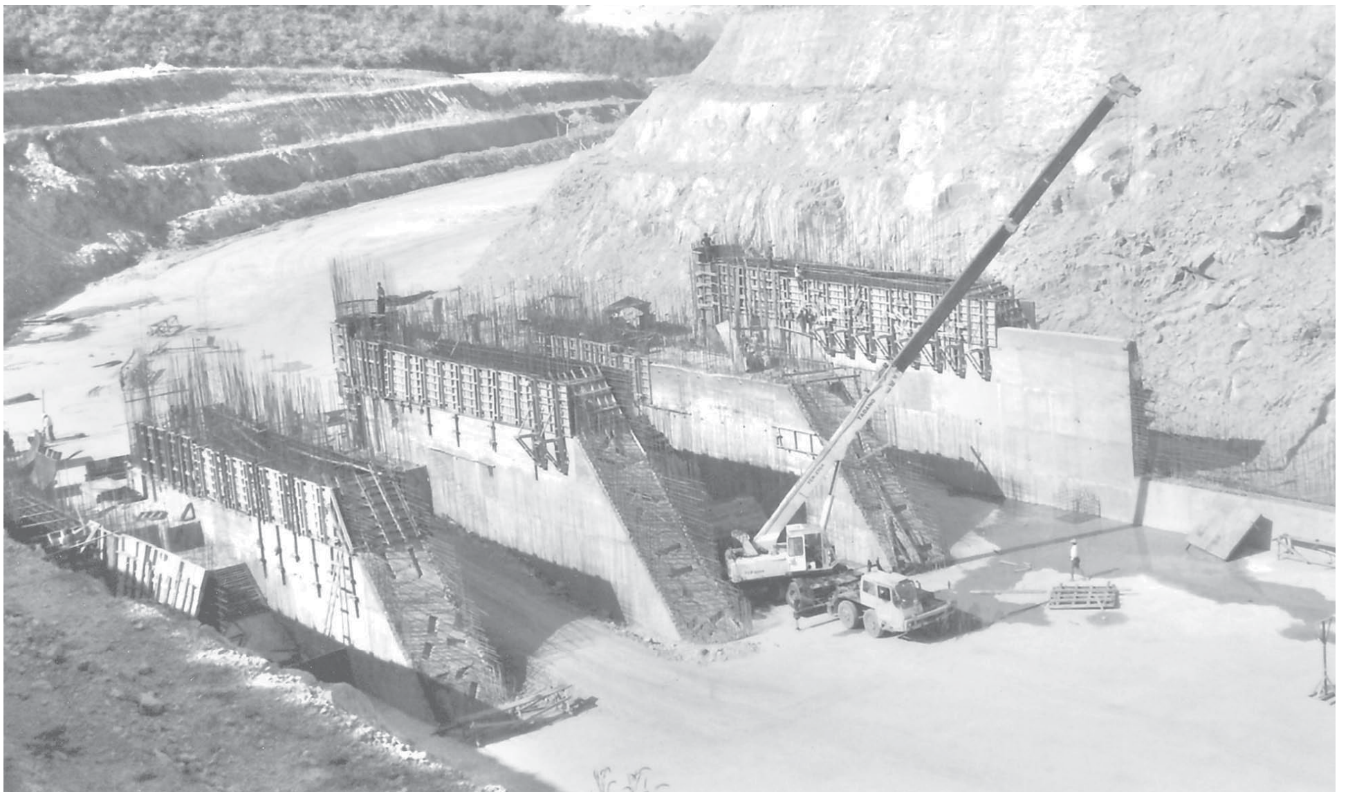
The three-gate spillway of Shwegyin Hydropower Project is under construction. — MNA
