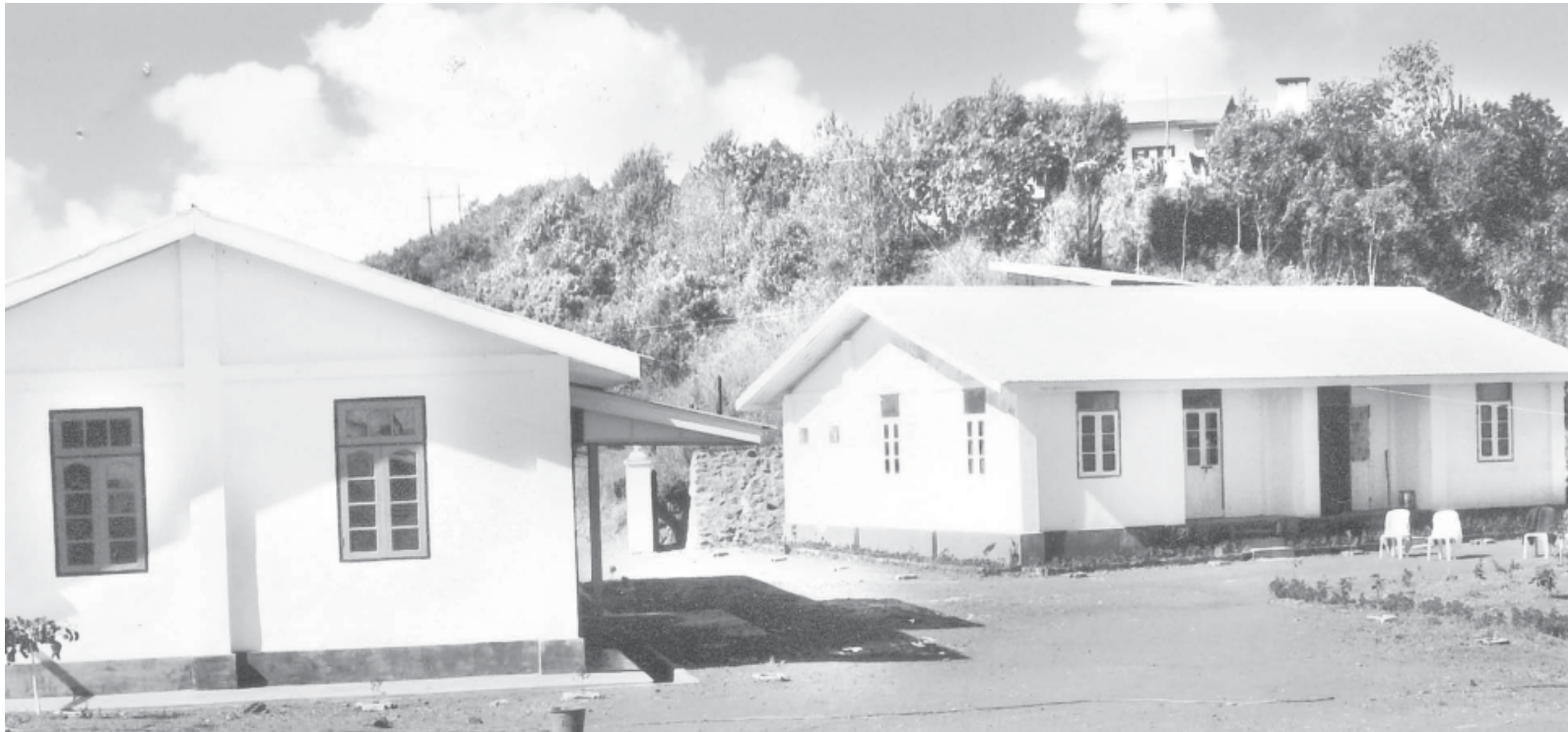
One storey hostel for trainees.
