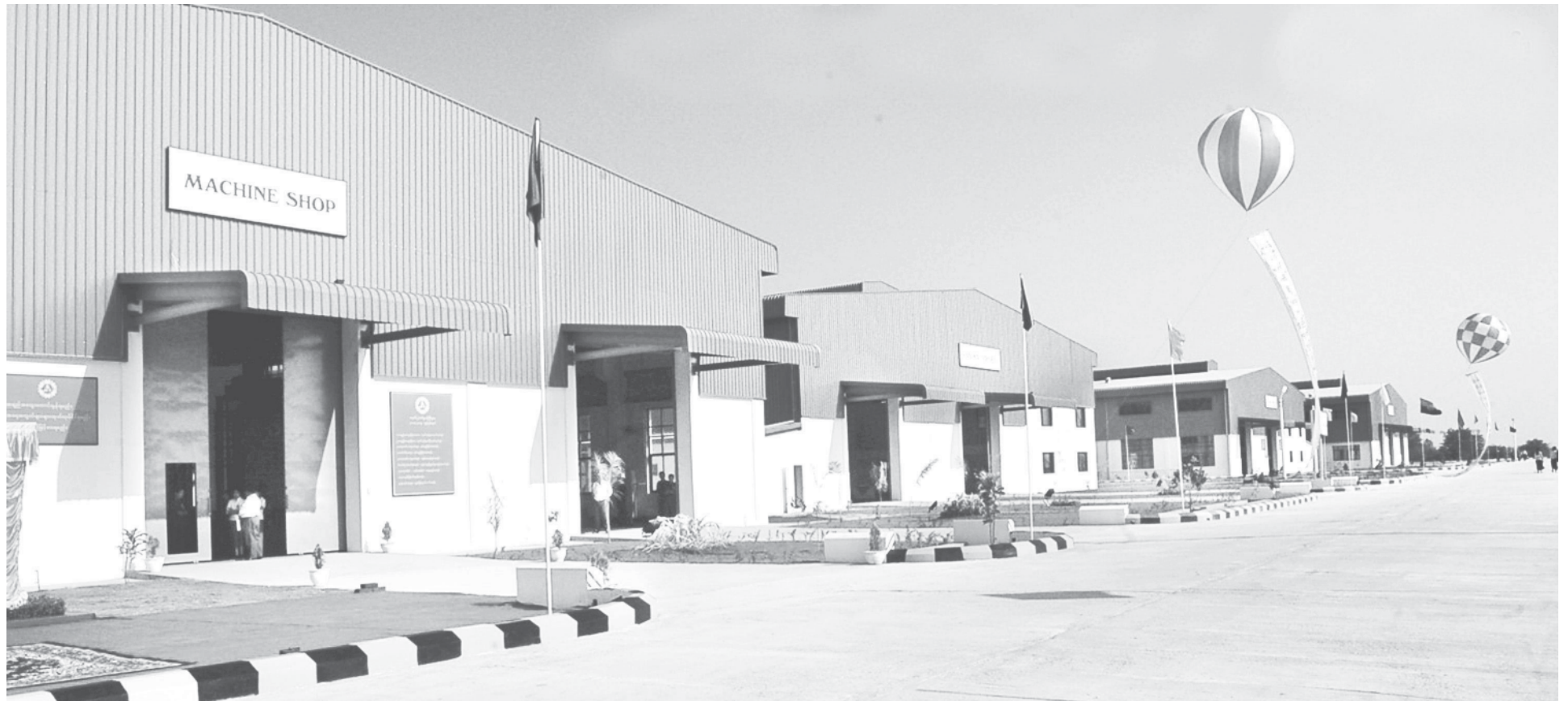
Machine and Machine Tools Manufacturing Plant (Myaing) of Ministry of Industry-2. (News on page 1)—MNA
