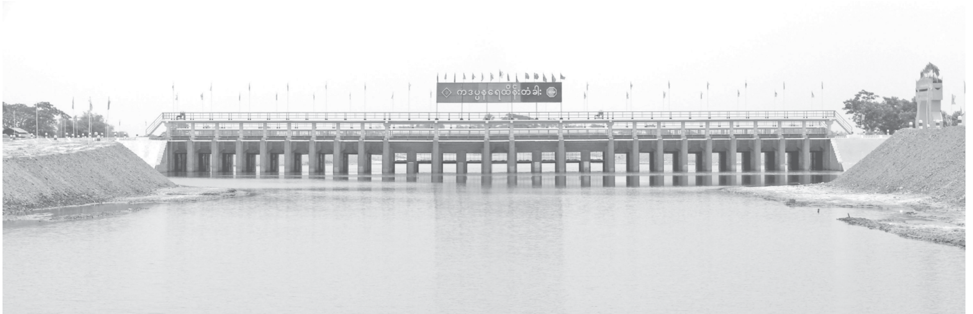
Kadapanna sluice gate constructed by Construction Group-6 of Irrigation Department near Kadapanna village in Kyauktan Township in Yangon Division.—MNA
