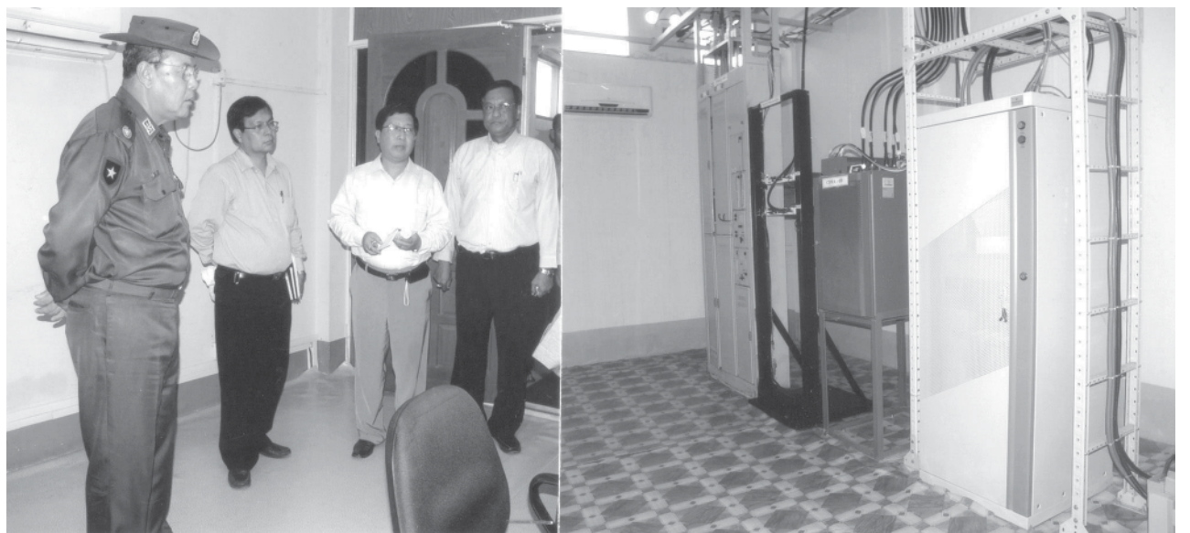
Minister Brig-Gen Thein Zaw inspects International Underground Cable Station in Pyapon.—MNA
