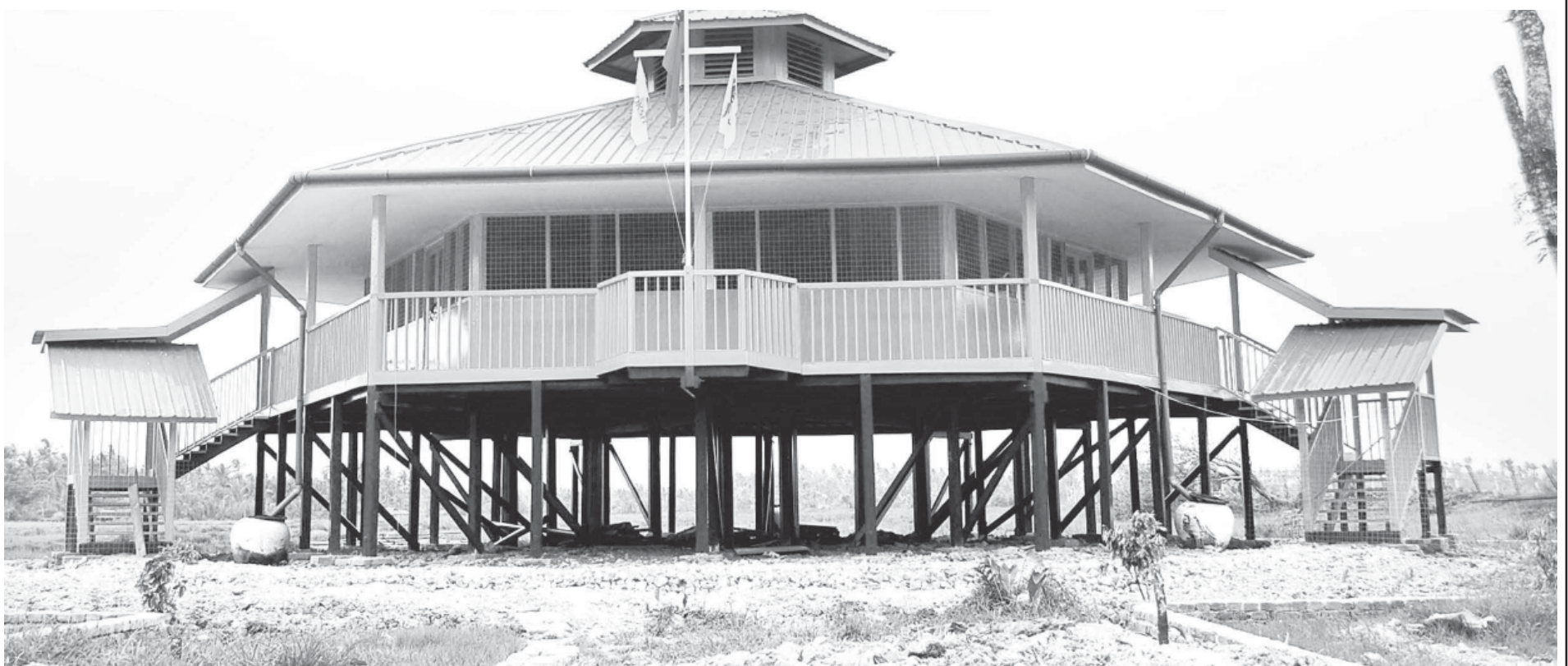
A Cyclone Shelter built near Taungthale Village of Bogale Township to accommodate local people.
