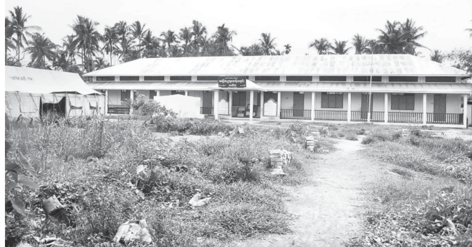
A BEPS constructed in Thabaung Village of Bogale Township as accommodation for local people in the event of a storm.
