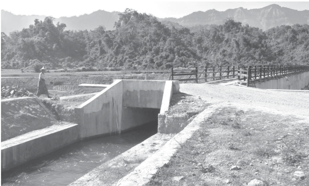
A bridge across a drain on motor road near Pyaingchaung Dam.
