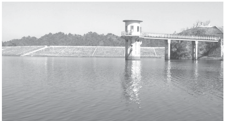
Water control tower of Pyaingchaung Dam.
