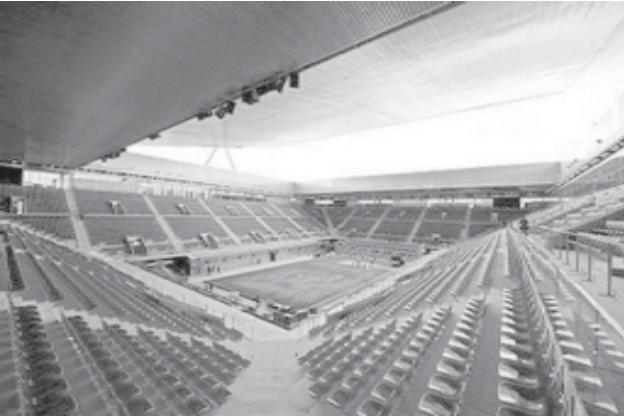
A view in Madrid of the Magic Box (La Caja Magica) arena by French architect Dominique Perrault, newly built to host the Madrid Combined Tennis Tournament which will take place from 8 to 17 May, 2009.— INTERNET
