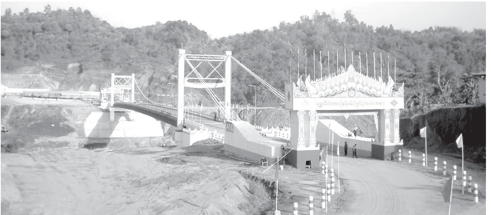
Photo shows Shweli Bridge (Namkham).—CONSTRUCTION
