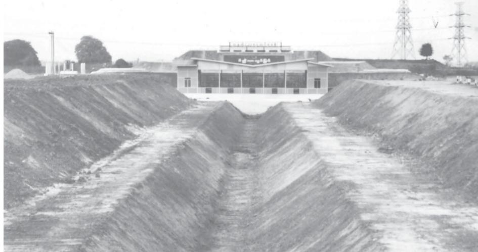
The photo shows the main canal under construction.
