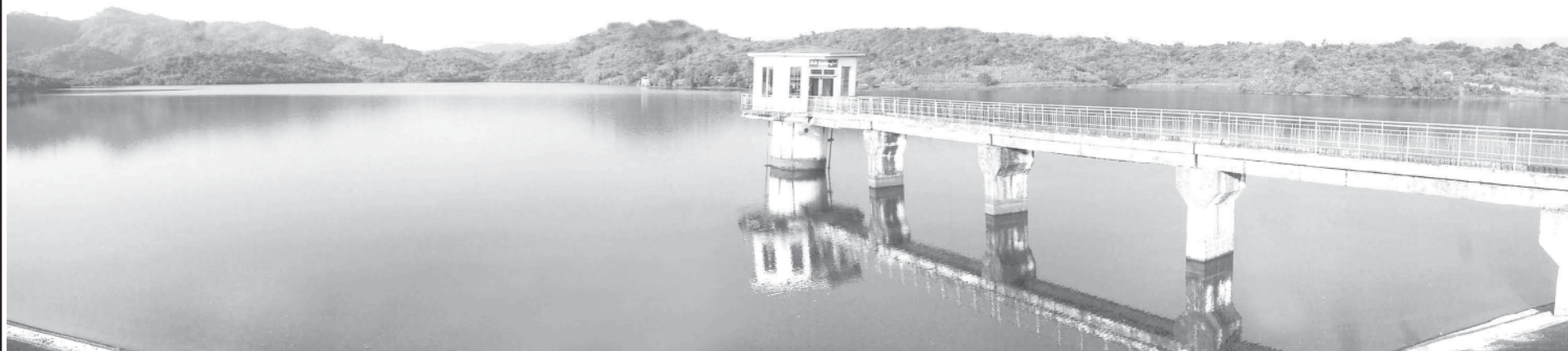
Wahpa Dam storing water for drinking water sufficiency of Thaton and for agriculture purpose of 2,400 acres of farmlands.
