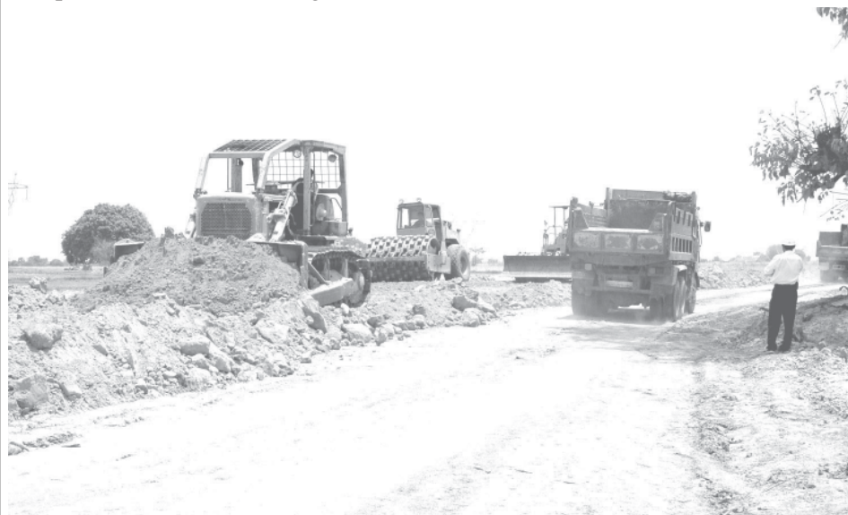
Roads under construction at Nay Pyi Taw International Airport.—MNA
