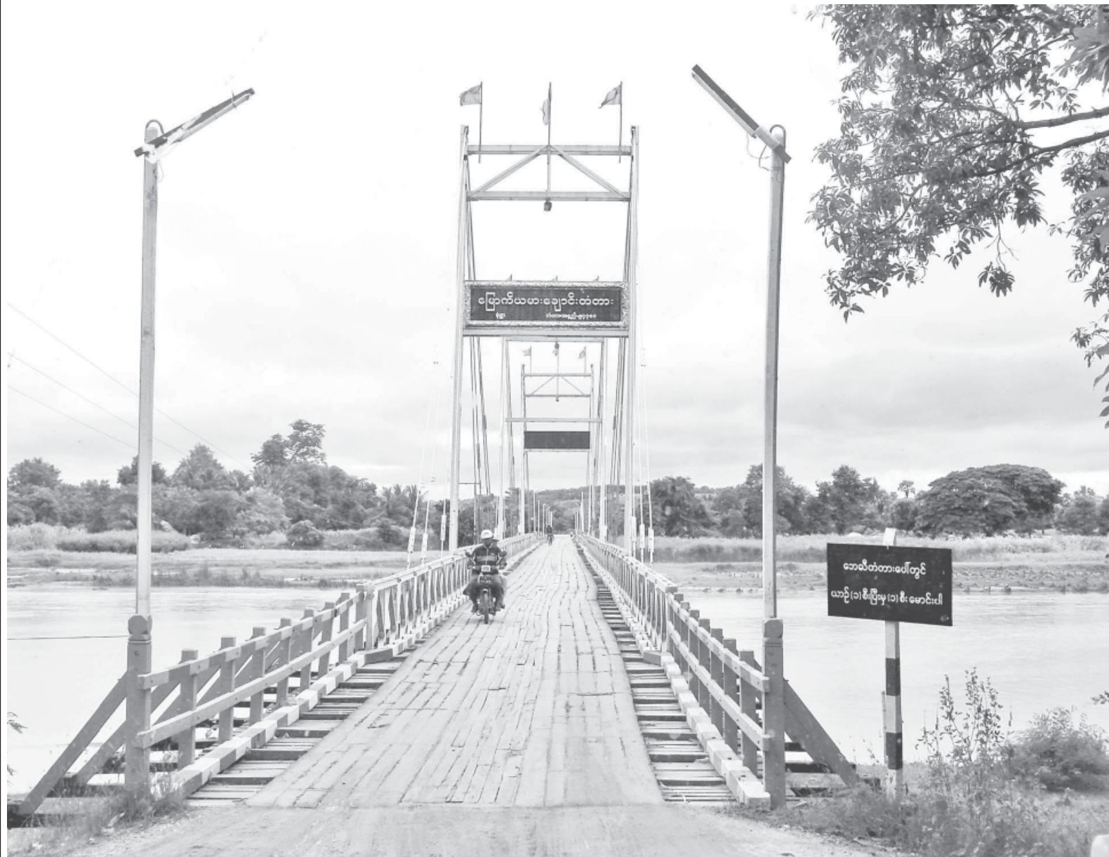
The wooden steel cable suspension bridge lies across North Yama Creek.
