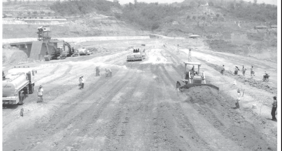
97 per cent completion of main embankment.
