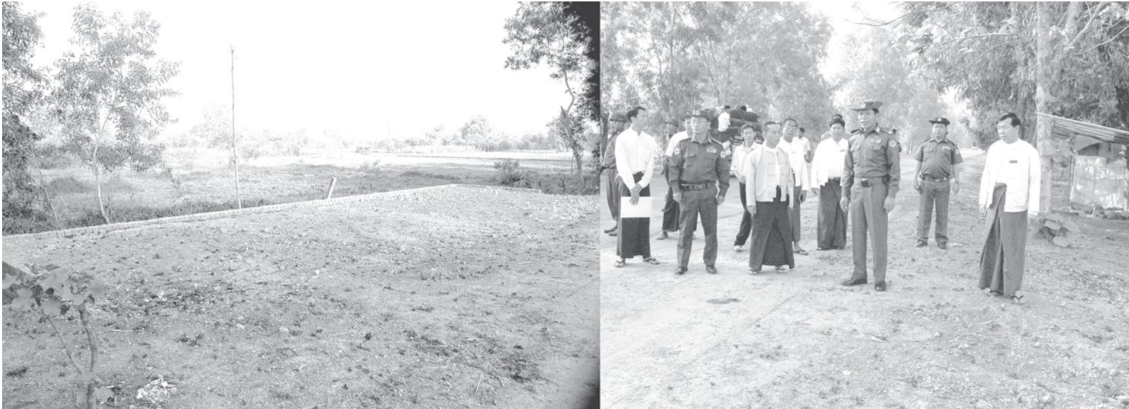
Commander Brig-Gen Win Myint inspects construction tasks of extended Yangon-Pyay road and designated places for the bus stops to be built.
