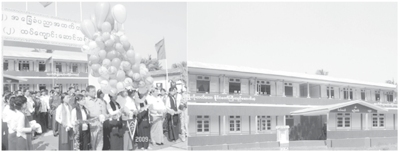
Commander Maj-Gen Kyaw Swe and Minister Col Thein Nyunt attend ceremony to open two-storey building for No. 2 Basic Education High School (Branch) in Maubin.—MNA
