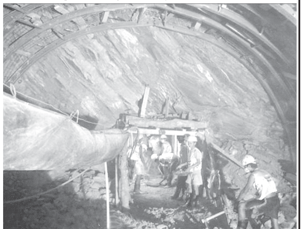
Workers and technicians drilling tunnel exit at Pyuchaung Hydropower Project.
