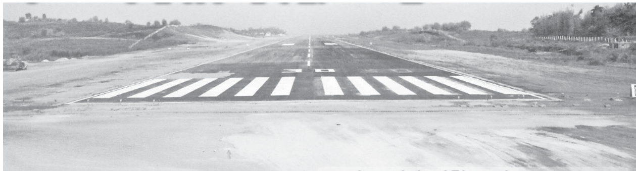
Photo shows newly-extended runway of Kengtung Airport.
