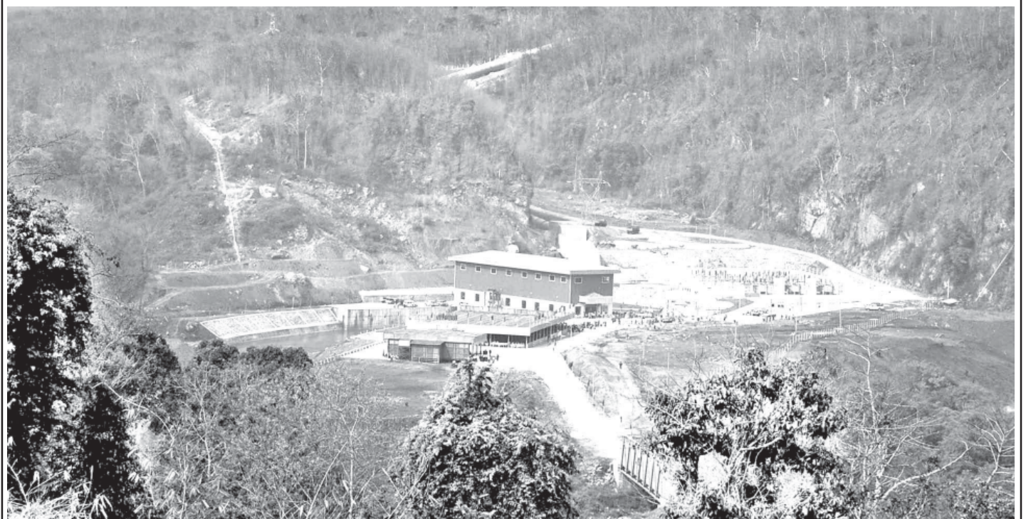
Kengtawng Hydropower Plant in Kengtawng region.
