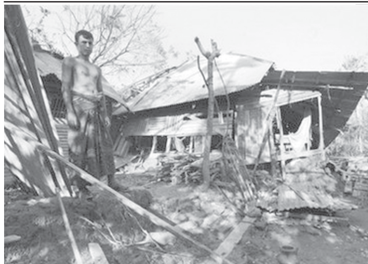
A cyclone packing winds of up to 90 kilometres (56 miles) an hour lashed Bangladesh’s southeastern coastal area, damaging houses and uprooting trees, officials said Saturday. INTERNET
