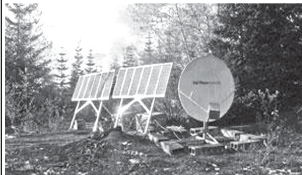
Scripps researchers installed an array of microbarometers at Mount St. Helens in November 2004 to collect infrasound near the site.
