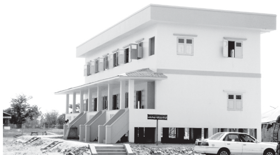
A Cyclone Shelter built in Thayetthonbin Village of Kungyangon Township.—ENERGY
