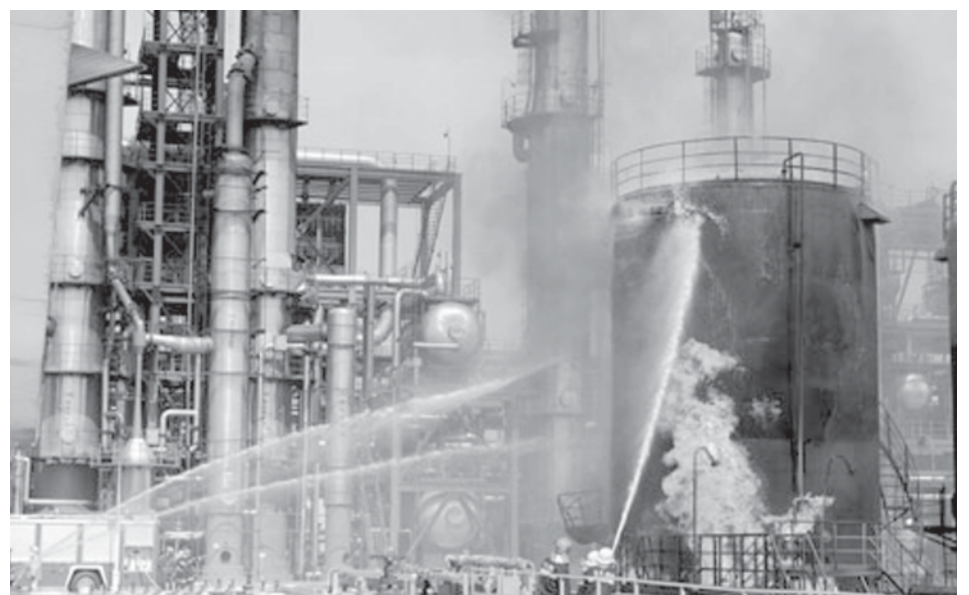
Firefighters hose down the fire at No 1 and No 2 light oil tanks of coal-to-liquids (CTL) projects base of Yitai Group in northwest China's Inner Mongolia Autonomous Region, on 8 April, 2009.—INTERNET
