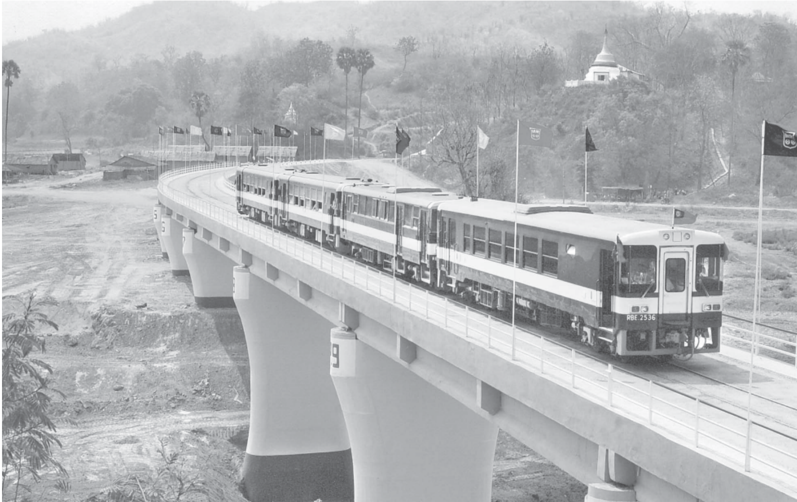
The 715 feet long Maday Bridge of Okshitpin-Kamma railroad section coping with the first train.
