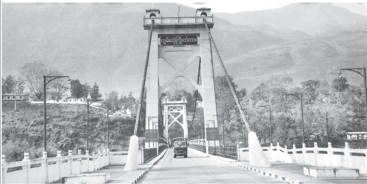
Kunlong Suspension Bridge on the Union Highway linking Yangon-Mandalay and Kyukok (Pangsai) and Muse is seen at the entrance to Kunlong, with the Shan Yoma mountain range in the background.
